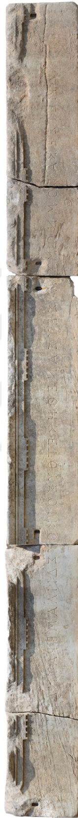
Figure 24 The architrave of the Oikoi building (O. Henry)
