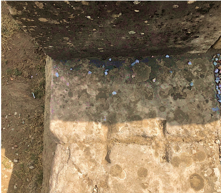
Figure 16 Dove-tail beddings on the stylobate (Ç. Durak)
