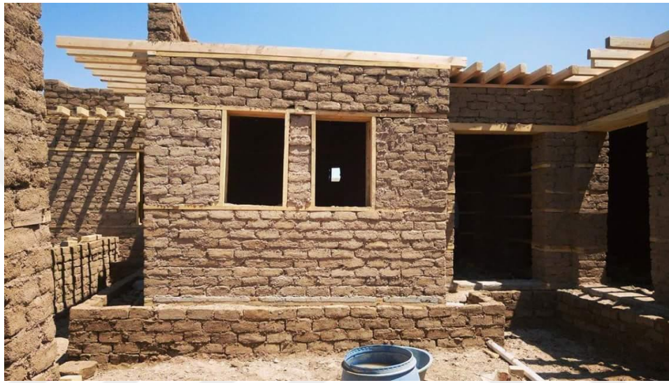
Fig.141: Using Beams for Roof Construction 49
