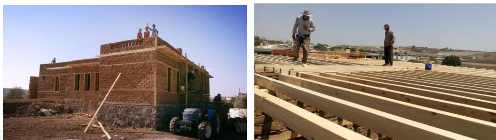
Fig.142: Roofing of a Mudbrick House 50
