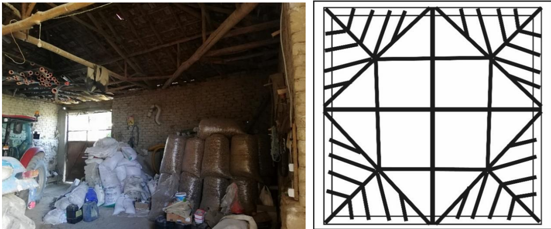
Fig.181: Roof Structure of a House from Kocayaka Village (Photo by M. Çarkı)
