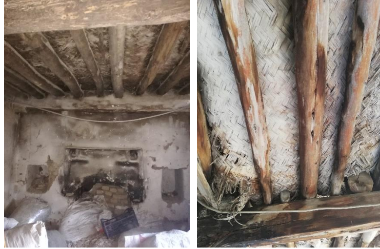
Fig.180: Kocayaka Houses Roof Sample (Photo by M. Çarkı)
