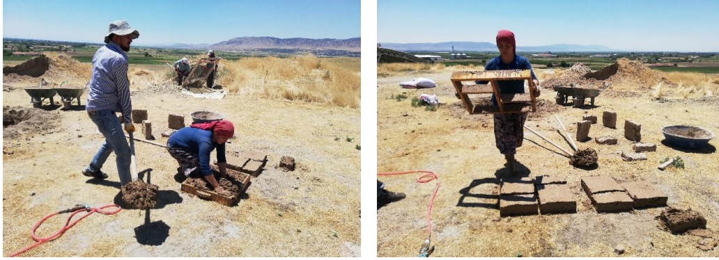
Fig.135: Mudbrick Mould and Pouring the Mudbrick to Moulds (Photo-M. Çarkı)
