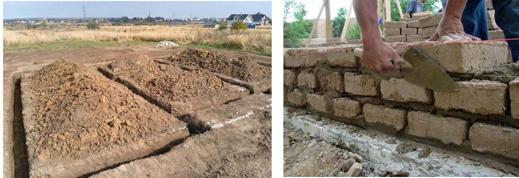
Fig.138: House Foundation 46 and Wall Construction 47
