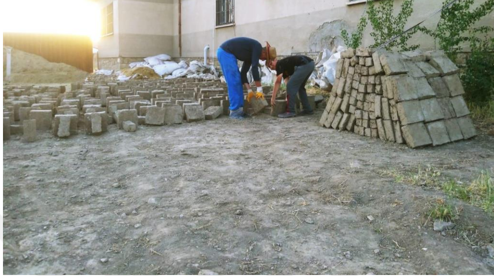
Fig.137: Dried Mudbricks and Stacking of Mudbricks 45
