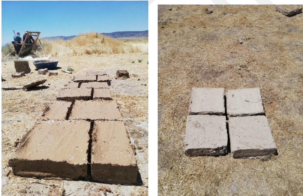
Fig. 136: Pouring the Mudbrick into the Mould for Drying (Photo-M. Çarkı)
