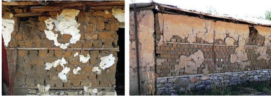
Fig.139: Stone Foundations and Wall Beams ( Photo-M. Çarkı )
