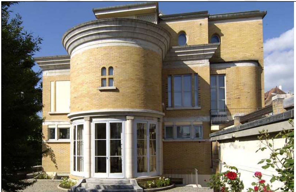
Figure 2.13: Villa Schwob (Foundationlecorbusier, n.d.b).
