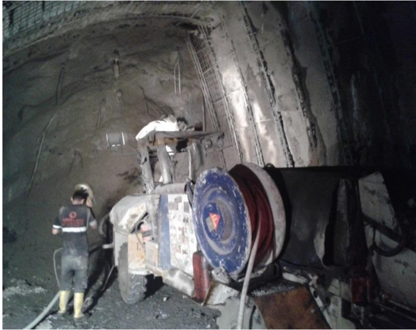
Figure 5.8: Shotcrete spraying machine and its application.
