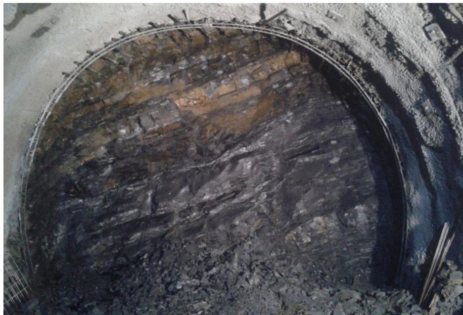
Figure 5.4: A photo of highly fractured tunnel face.
