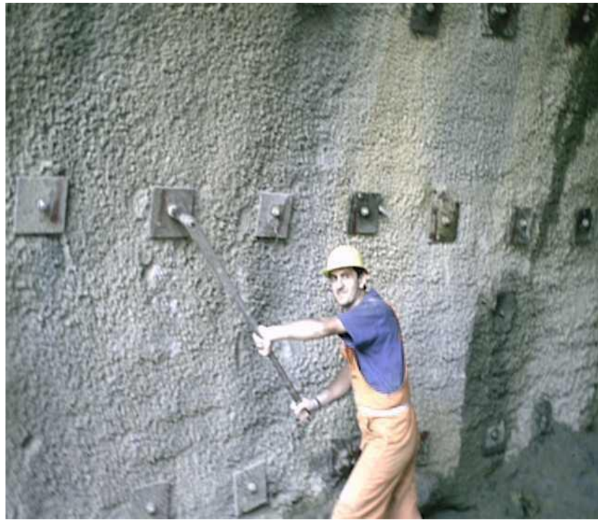
Figure 5.6: Torque application on bolts.
