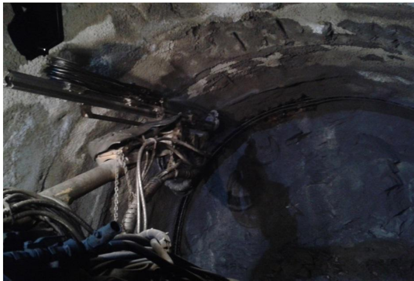
Figure 5.10: Spile application.
