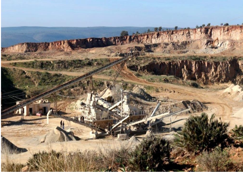
Figure 3.17. Overview of limestone crushing plant at the level of the Q5.
