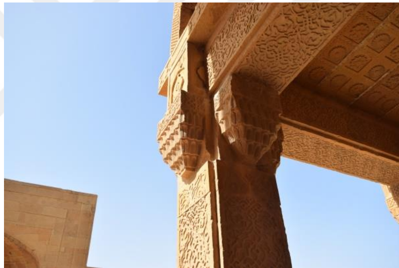
Figure 53: Corner visual of the four bracketed capitals and post and lintel arabesque moldings, Tomb of Isa Khan Tarkhan II.
