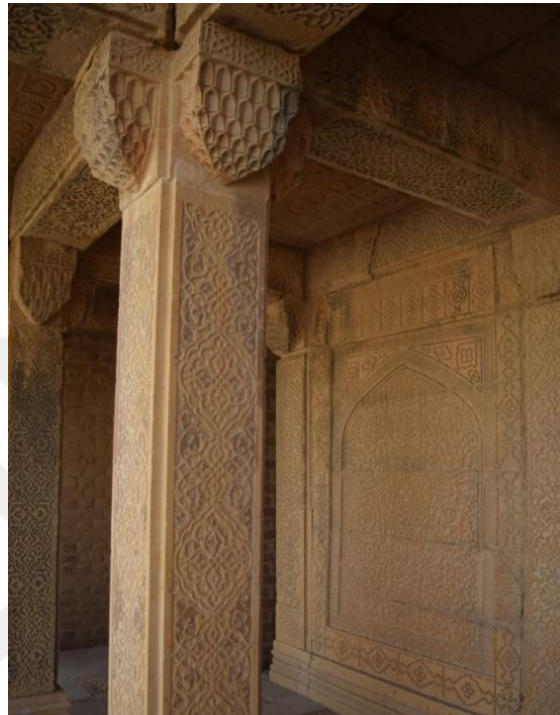
Figure 51: Arabesque details of the column with four bracketed muqarna capitals, Colonnade of Tomb of Isa Khan Tarkhan II
