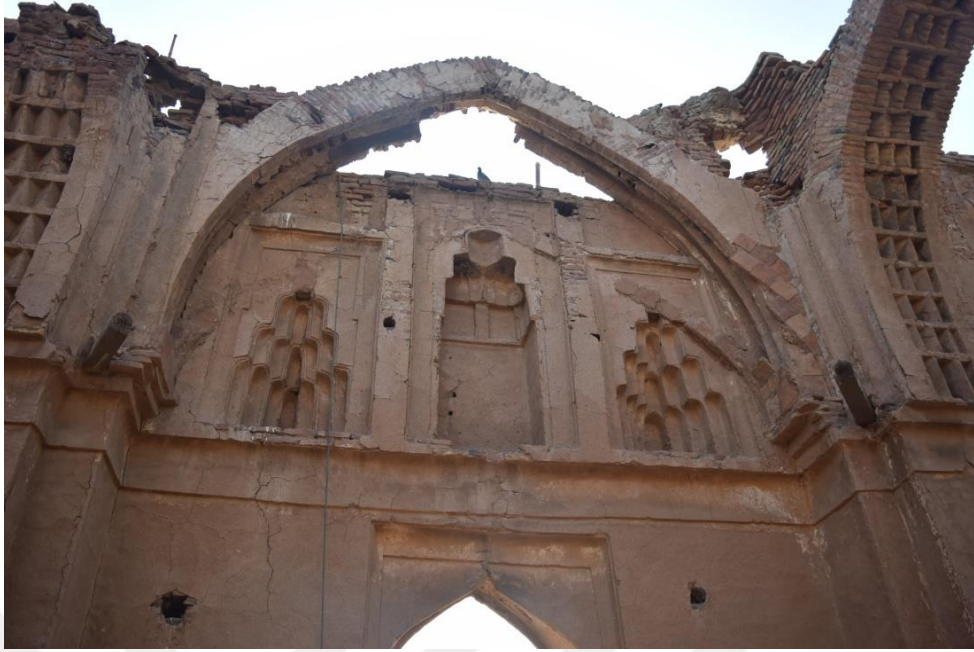
Figure 71: Muqarna/ stalactite moldings in the interior of Makli Masjid (1389-92 CE), Samma Period.
