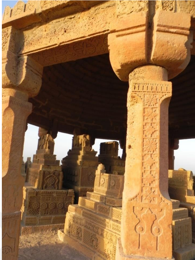
Figure 105: Canopy Pavilion and bracketed columns, Chaukhandi.
