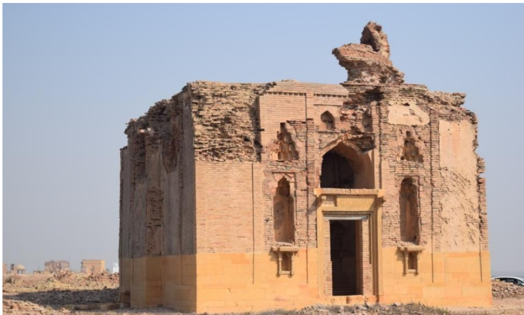
Figure 67: South west view indicating remains of plaster and dentils, Kaus Sultani (1513 CE), Samma Period.
