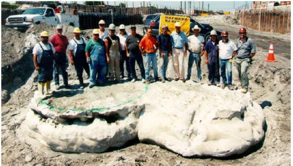
Figure 5.17 Columns created with the Super Jet Grout Method
