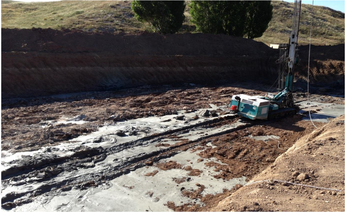
Figure 5.10 Injection stage
