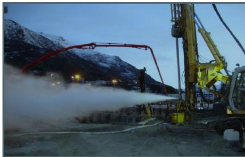
Figure 5.9 The water used in drilling process (Kimpritis, T, 2013)
