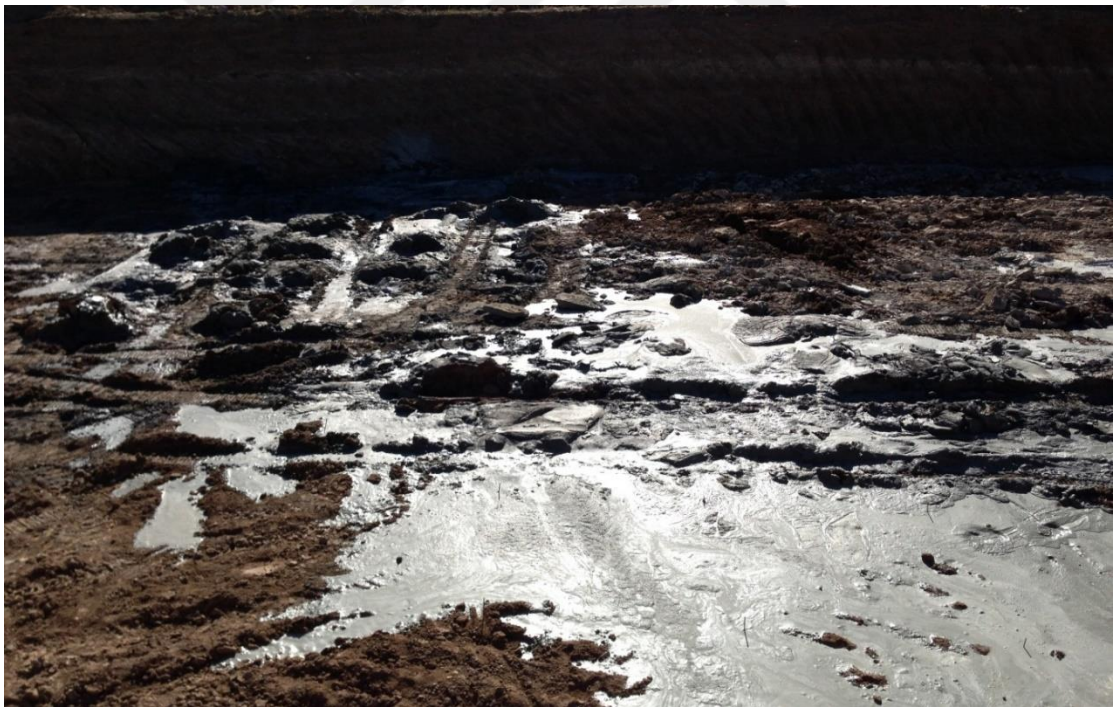
Figure 5.11 An image of the jet grout application after the injection
