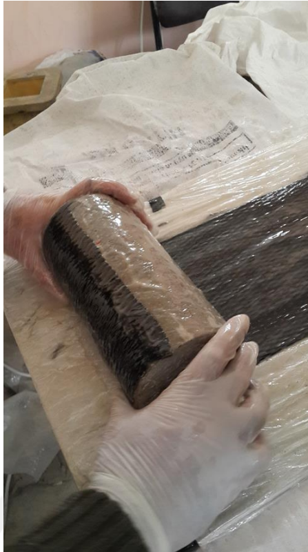
Figure A9 Initial step of application the FRP fabrics
