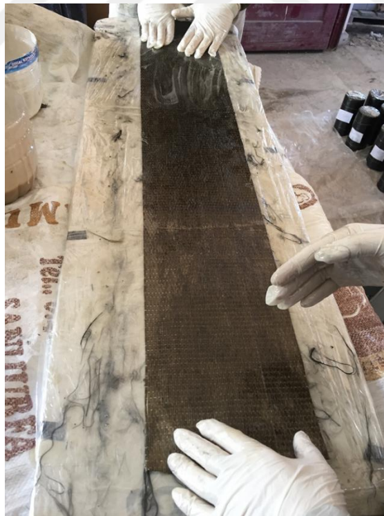
Figure A8 Preparing the FRP sheet
