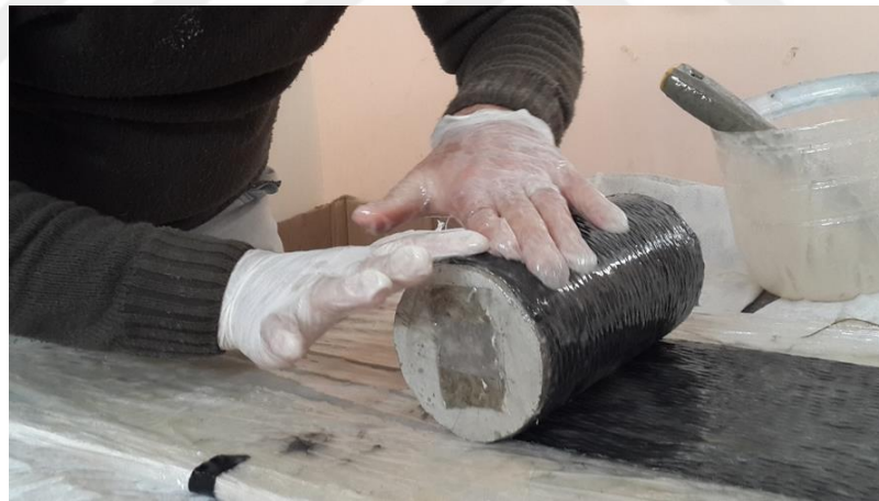
Figure A10 Continue the application of FRP fabrics
