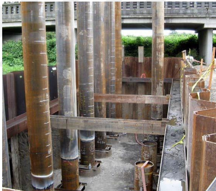
a) CFST pile groups supporting the main span of the Nooksack River Bridge
