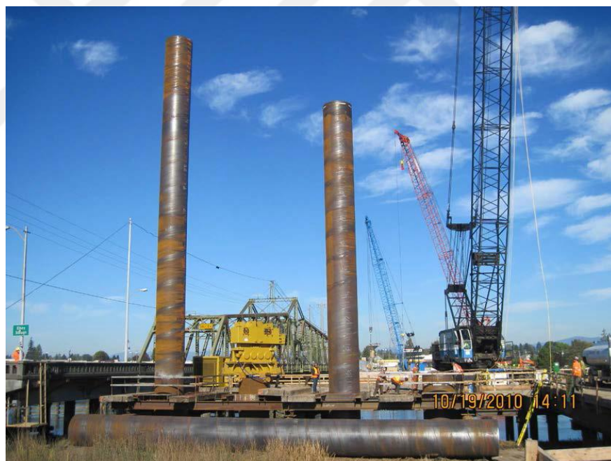
a) Pile driving on the Ebey Slough Bridge
