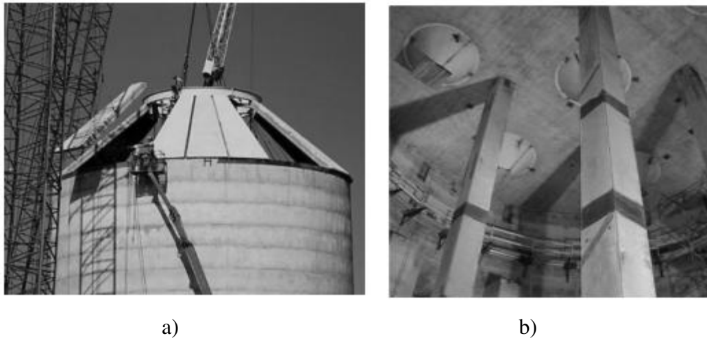
Figure 2.4. UHPC construction examples: (a) UHPC panels on Joppa clinker silo and; (b) 54 ft UHPC columns in Detroit [69]
