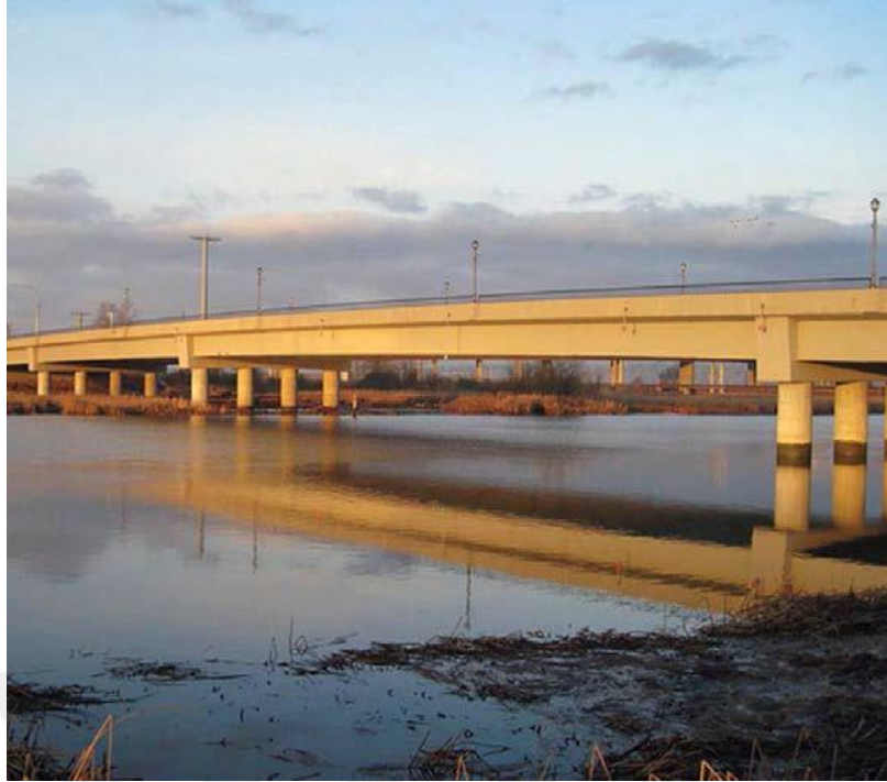
b) Completed Ebey Slough Bridge
