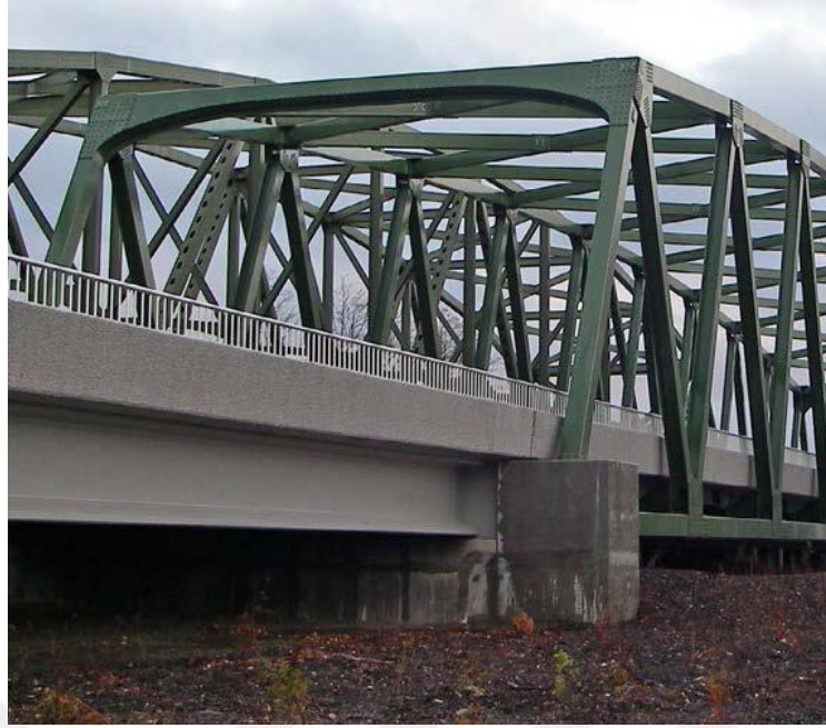
b) Completed Nooksack River Bridge
