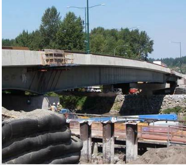
b) Completed Puyallup River Bridge
