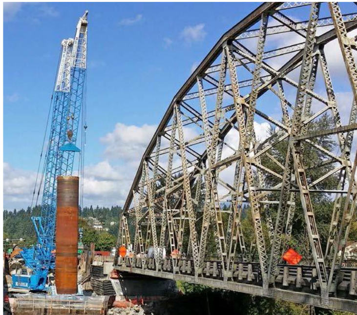
a) Shaft installation on the Puyallup River Bridge
