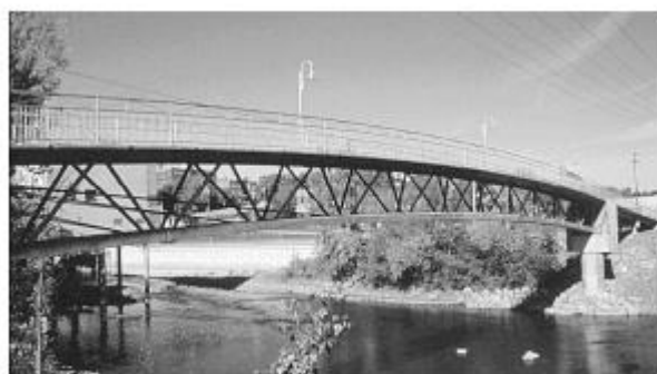
Figure 2.2. UHPC example: Sherbrooke footbridge [72]
