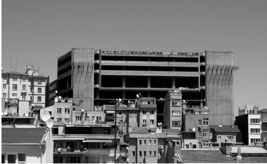
Figure 3. 11. A recent photograph of Park Hotel as seen from the Bosphorus (Photograph by Metehan Özcan).
