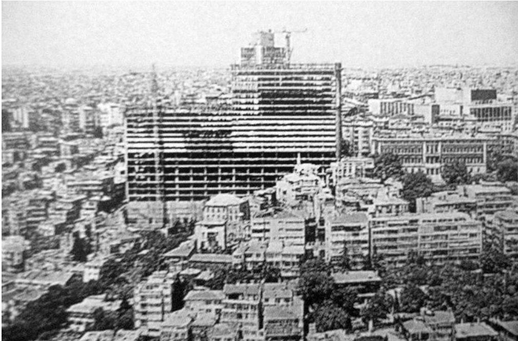
Figure 3. 9. The New Park Hotel construction before its excessive stories were slashed (Gökdağ, 1992).
