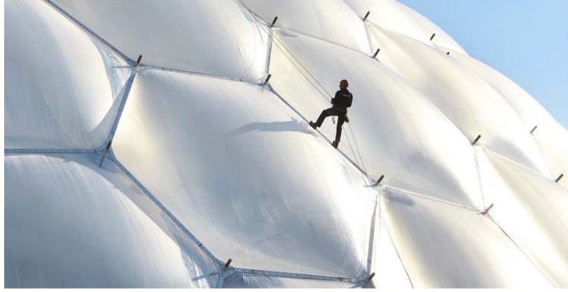
Şekil 35: (Ethylene-Tetrafluoroethylene Copolymer) ETFE paneller
