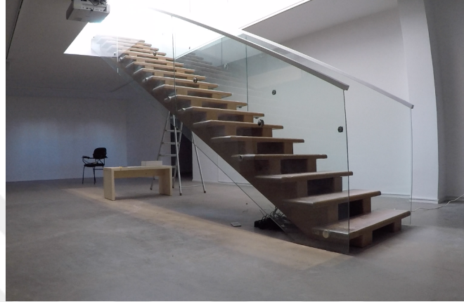
Figure 3.4: 10 transducer speakers attached to the stairway
