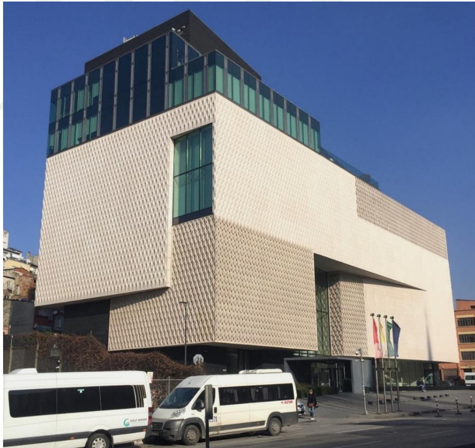
Figure 4.24 Arter's View from the Irmak Street
