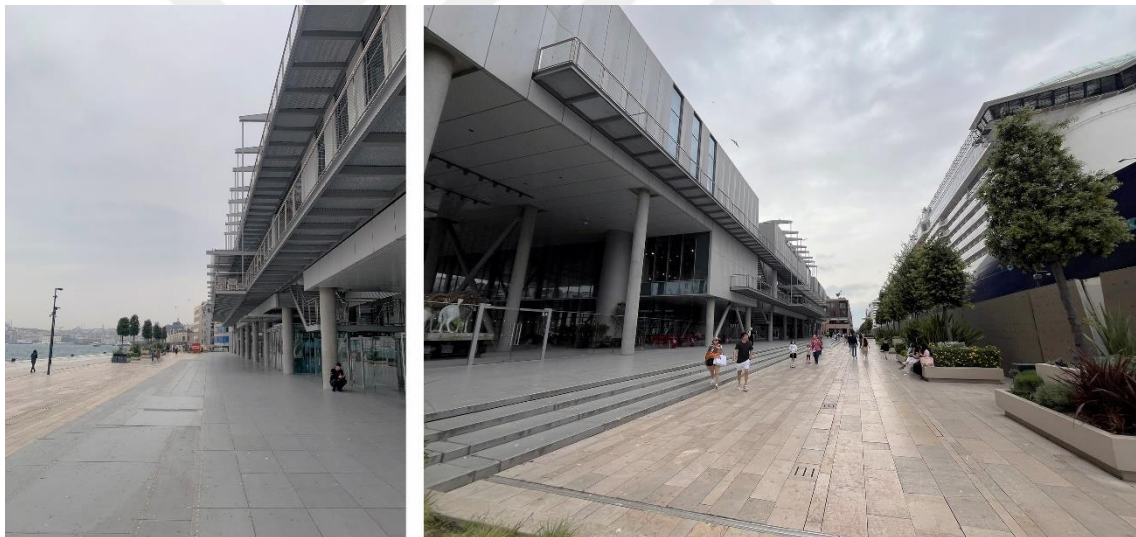
Figure 4.15 The Pedestrian Path in Front of the Museum: Normal and Raised States of the Dock
