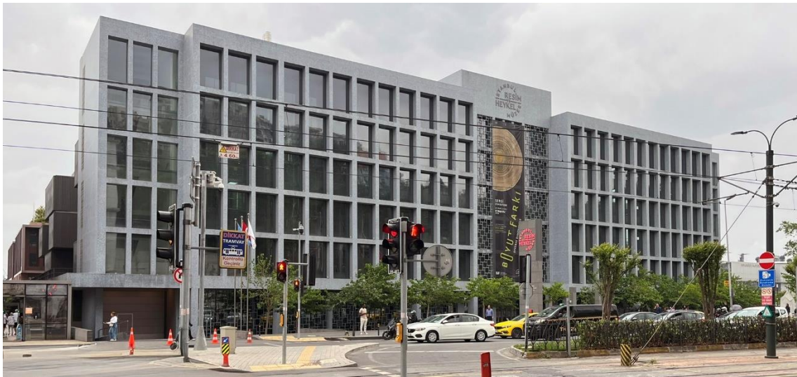
Figure 4.3 IMPS Street Side View
