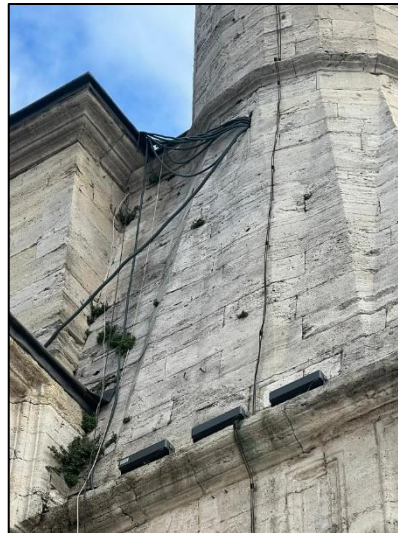
Figure 5.16: Separation Formed in Yeni Camii.
