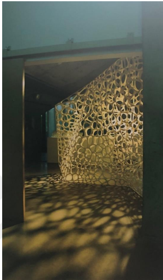
Figure 4.23: C Wall (38) demonstrating Packing Parametric Design Pattern (Iwamoto, 2009: 85)
