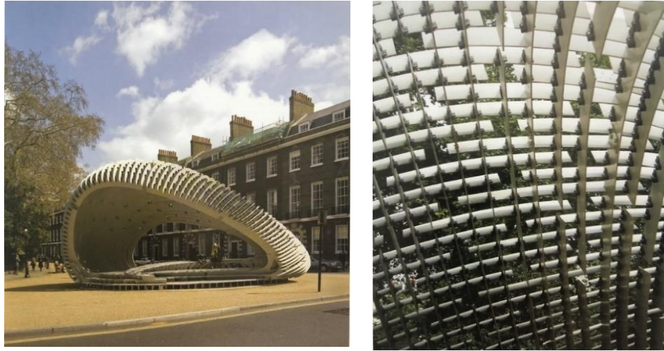
Figure 4.24: Interlocking cross joint system of (c) Space (4) as Weaving Parametric Design Pattern (Krauel 2010: 30, 31)
