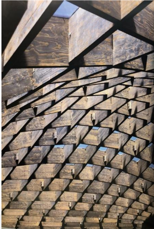
Figure 4.9: Mortise-tenon connection of Serpentine Gallery Pavilion (3) (2005) by Alvaro Siza and Eduardo Souto de Moura (Alvaro Siza and Eduardo Souto de Moura with Cecil Balmond, 2005: 100)
