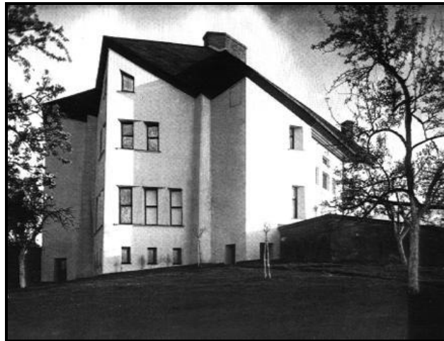
Şekil 3.4 Wylerberg Evi, Kranenburg (Niederrhein), 1921–24 mimar: Otto Barning
