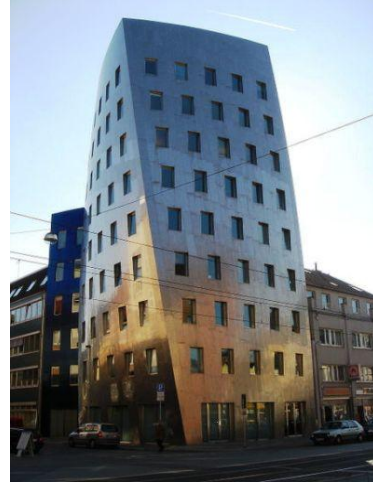
Resim 3.6. Ustra Building Office[22]
