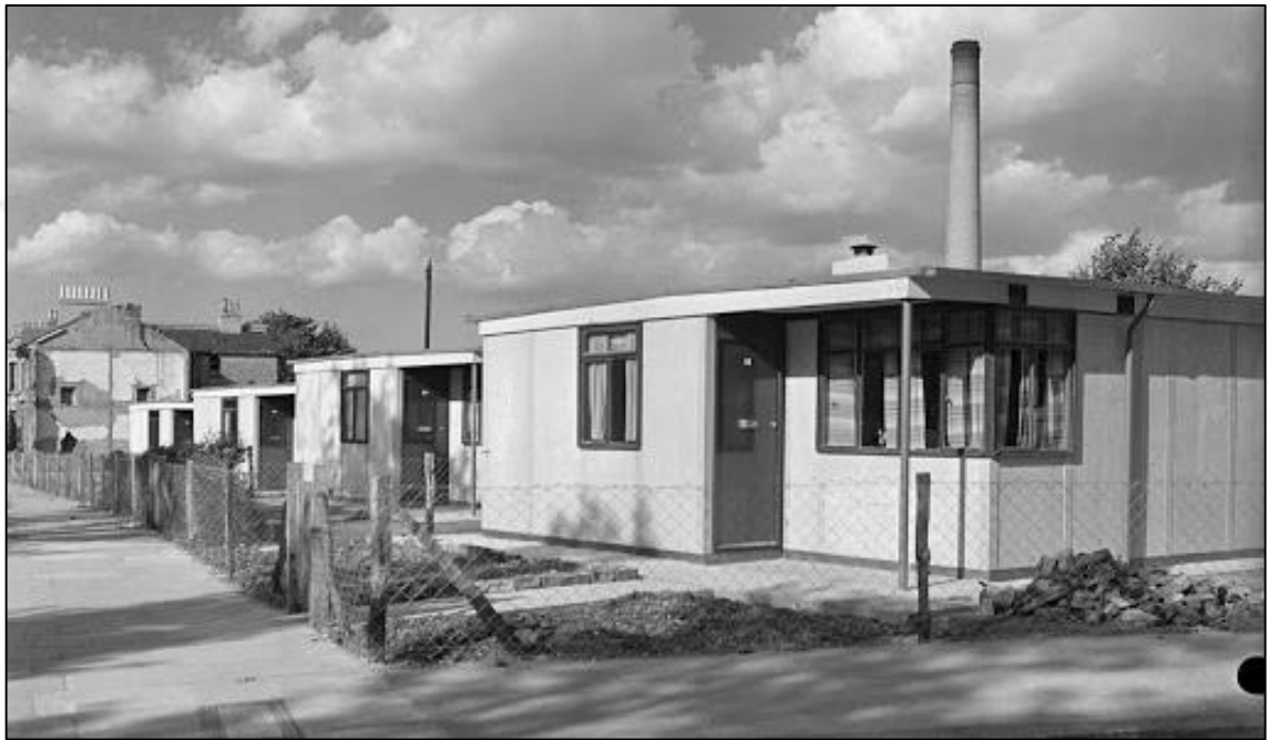
Figure 2.5. Uni-Seco prefabricated houses, London [22].
