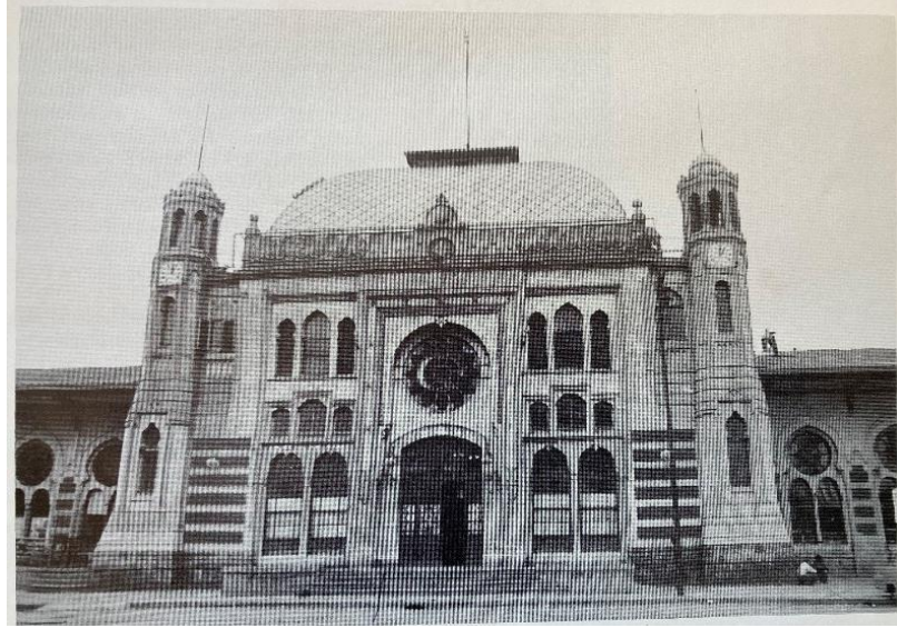
Figure 35 - Sirkeci Railroad Terminal, Istanbul, (Jachmund, 1890). Source: Modern Turkish Architecture (1984)
