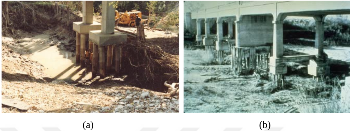
Figure 2.7. Examples of (a) uniform scour (Abd El Samee & Elsamny, 2019) (b) non-uniform scour (USGS)
