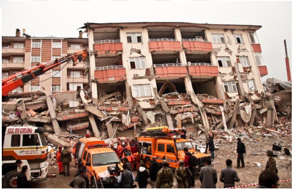
Figure 1.3 Building had collapsed 2011 in the earthquake (Taken from the archive of Assoc. Prof. Dr. İdris Bedirhanoğlu, Bedirhanoglu 2011b)
