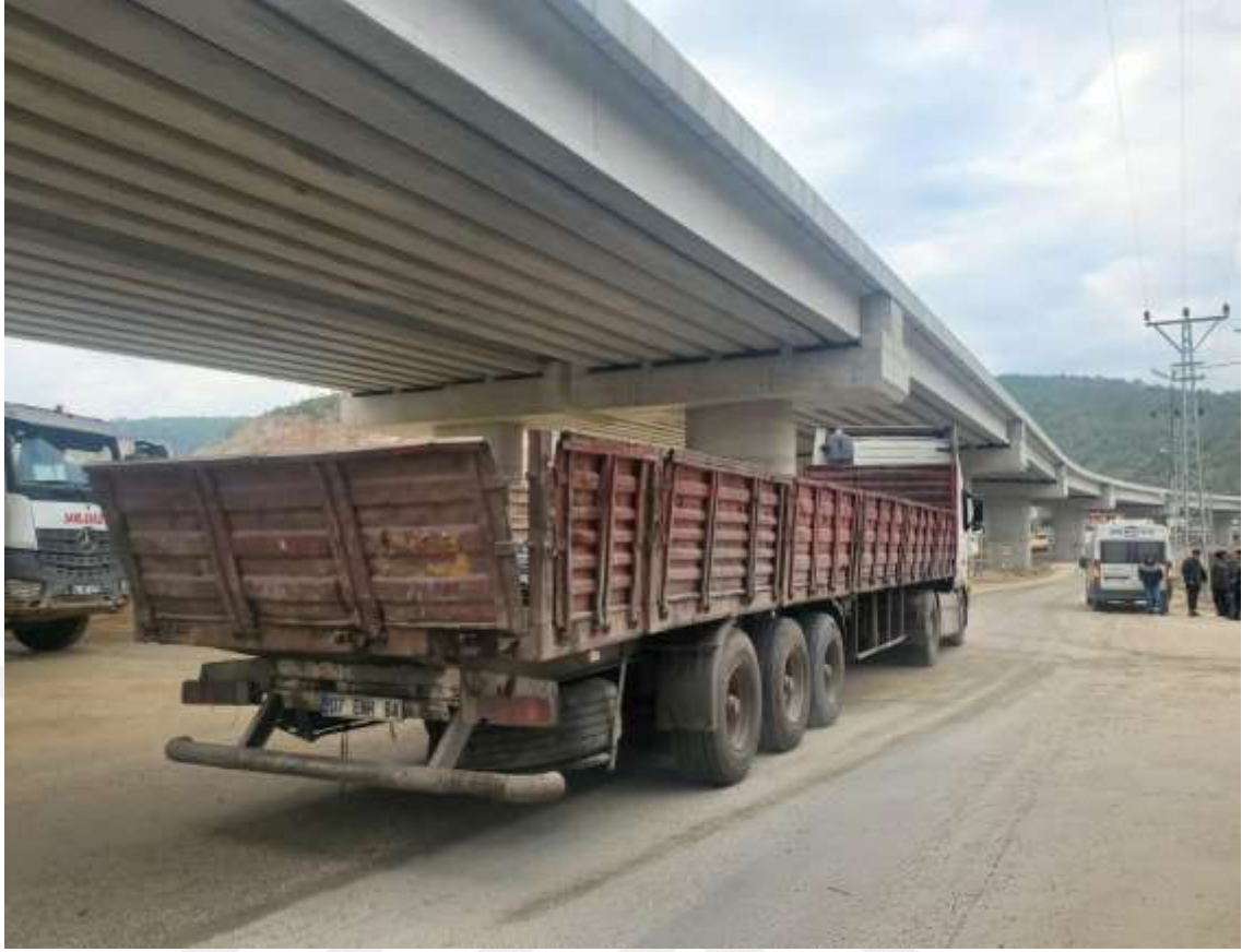
Figure 7. Trucks and the new viaduct in Büyükeceli
