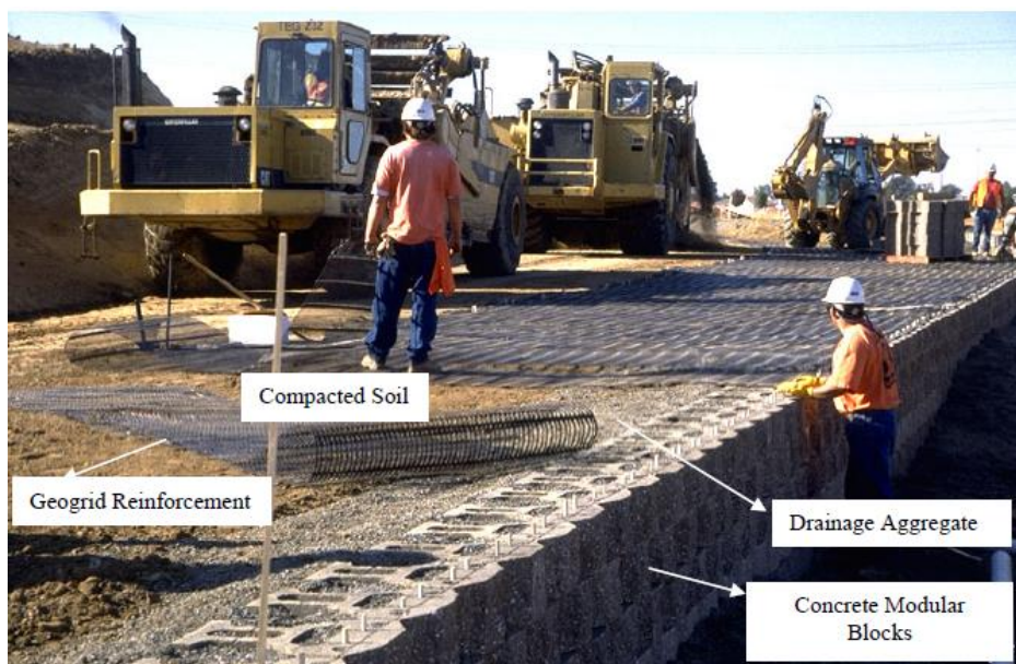
Figure 2.3. Construction process of a Geosynthetic-Reinforced Soil Structure [10].
