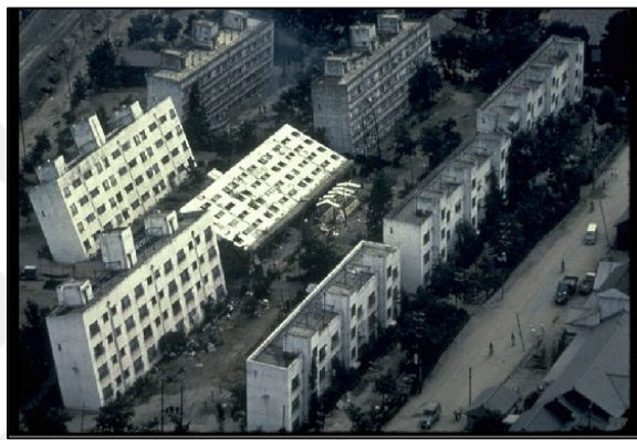
Figure 1.3: Tilting Of Apartment Buildings Caused By The 1964 Niigata Earthquake (Photo: National Information Service for Earthquake Engineering, EERC, University of California, Berkeley).
