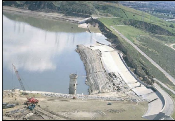
Figure 1.4: Lower San Fernando Dam After The San Fernando Earthquake (1971). (Courtesy Of The National Information Service For Earthquake Engineering, EERC, University Of California, Berkeley).
