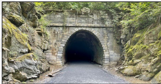
Figure 1.12: Elliptical Shape Tunnel.
