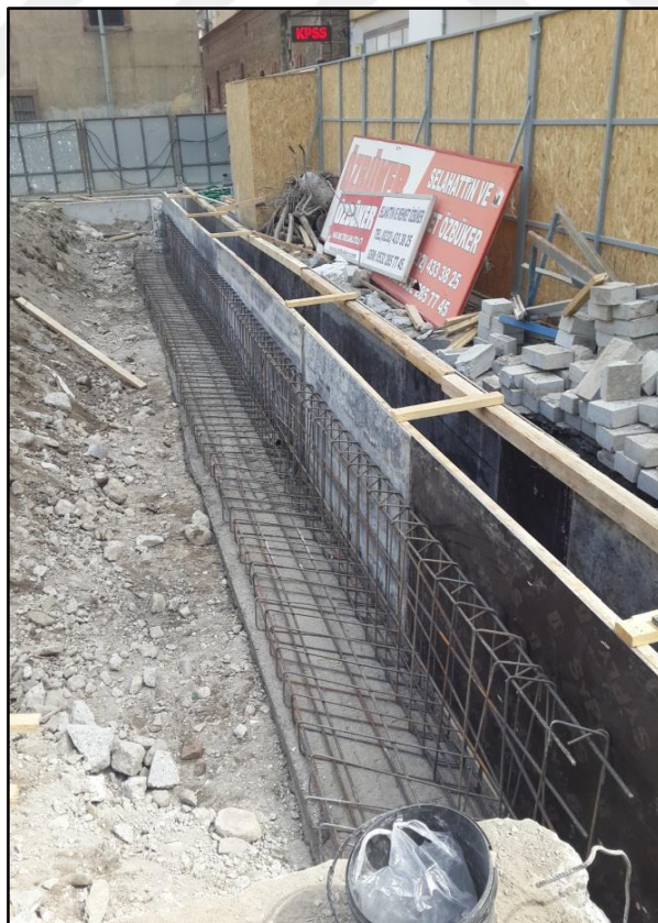
Figure B.2 Preparing the guide wall - 2
