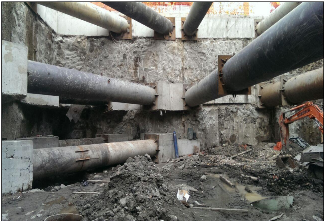
Figure B.8 During excavation stage-2
