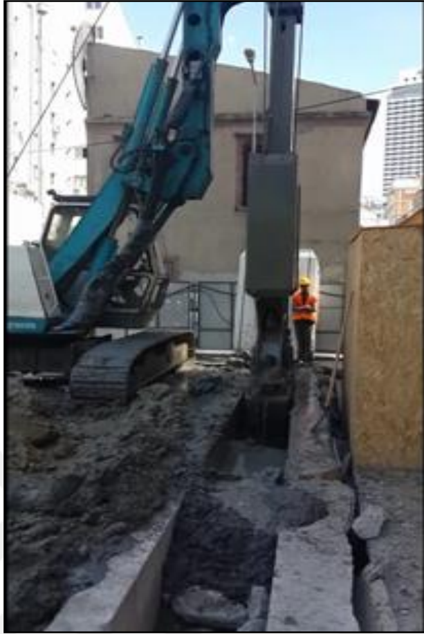
Figure B.3 Trench excavation
