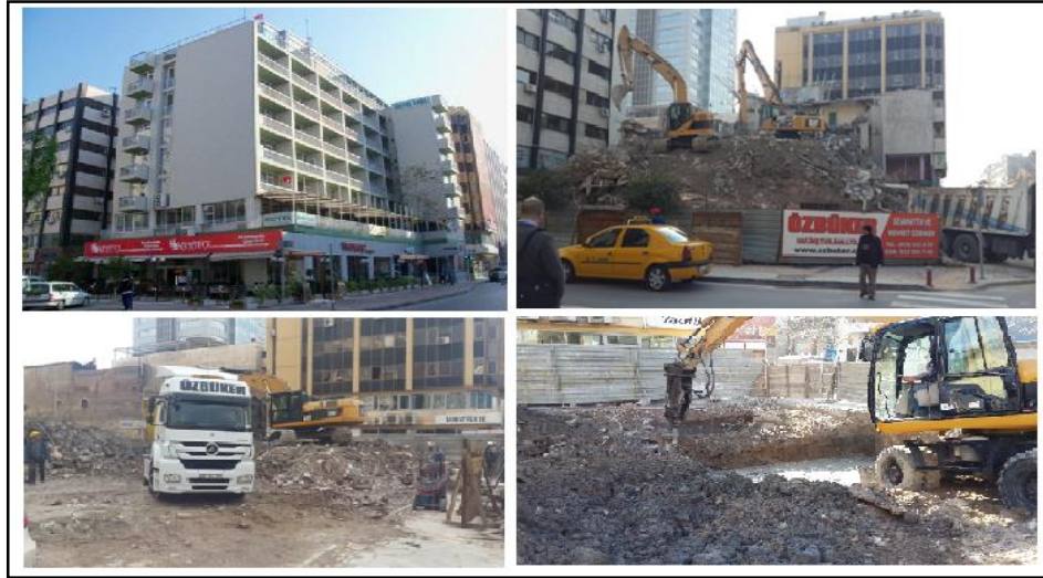
Figure 3.2 Existing building, Anba Otel and its demolition
