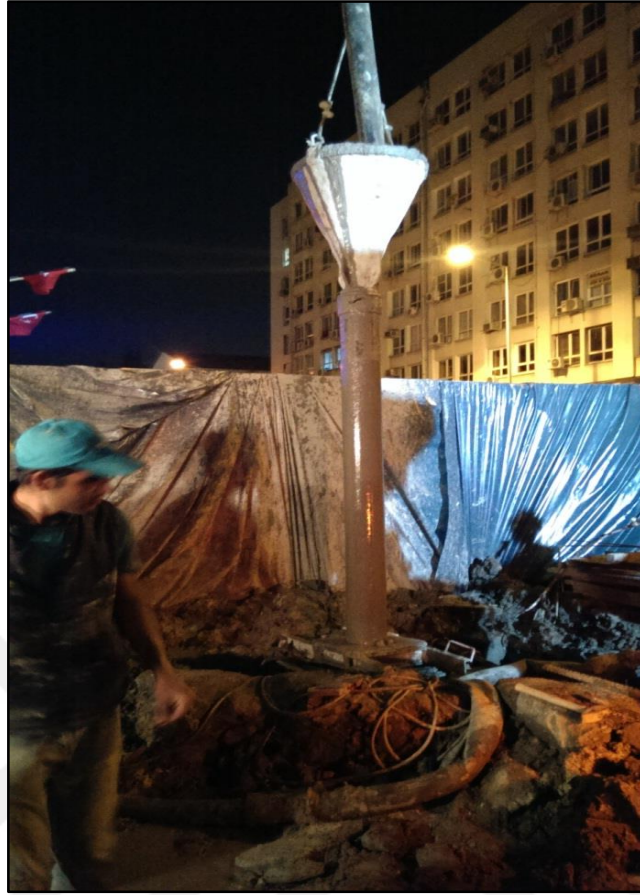
Figure B.5 Concreting stage
