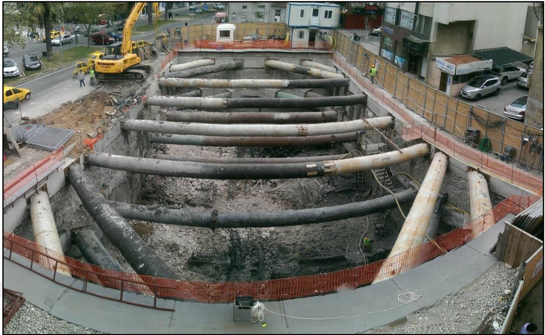
Figure B.7 During excavation stage-1
