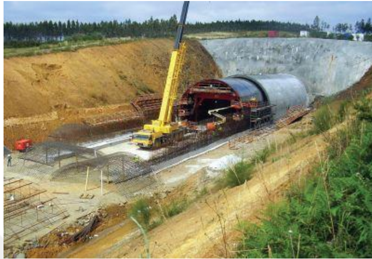
Figure 2.11. A Site View of the Cut-and-Cover Method in Practice (adapted from Infrastructure Construction Archives, 2020).
