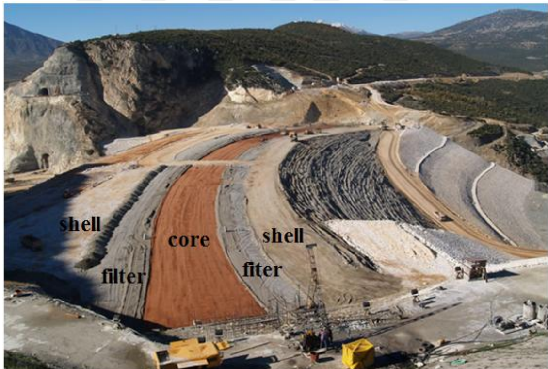
Figure 2.8. A zoned earthfill dam under construction(Source: Web_4 2015)
