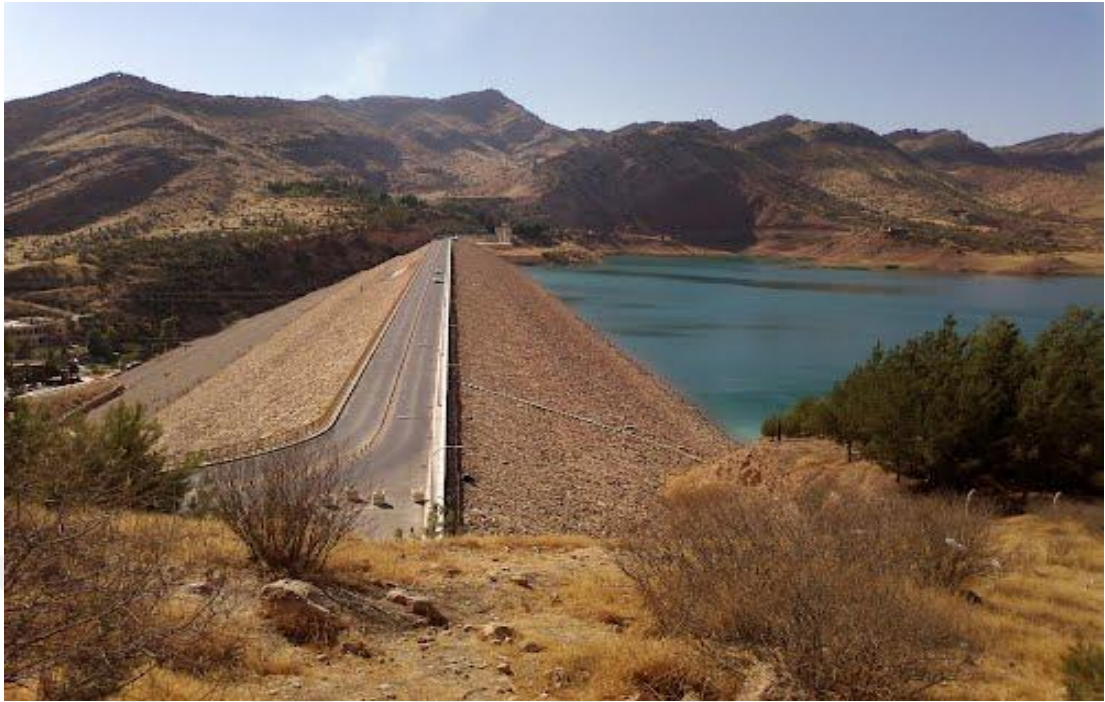
Figure 2.5. Duhok Earth dam.(Source: Web_3 2015)
