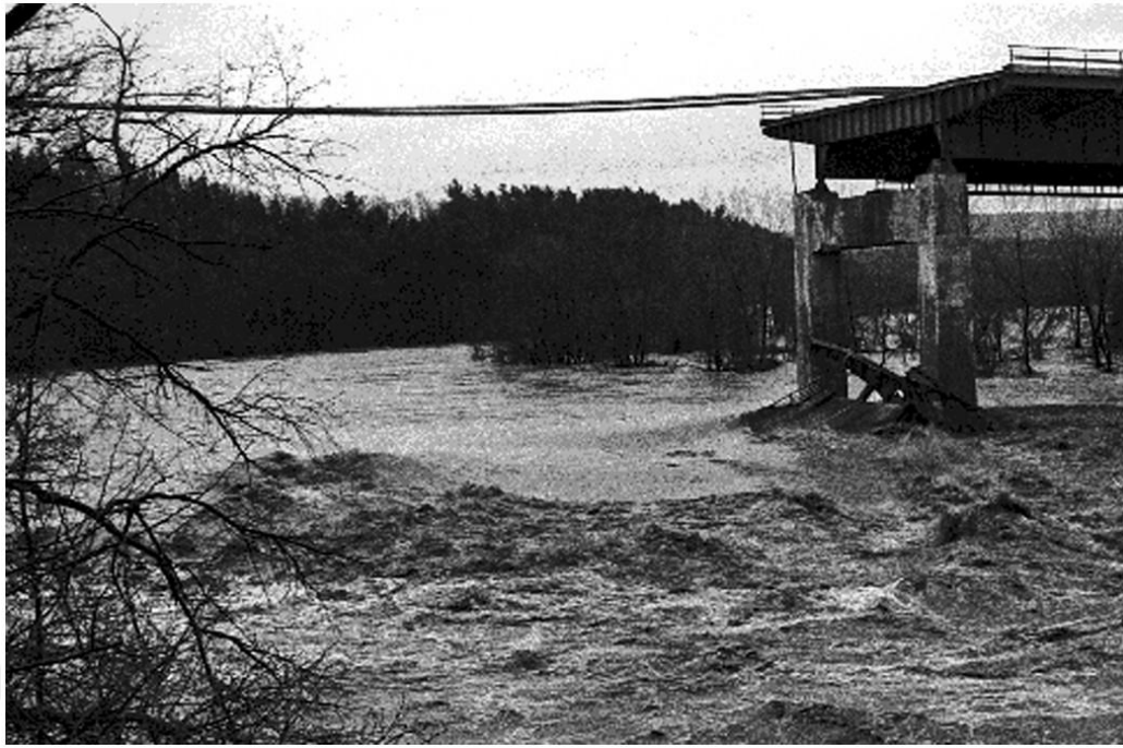
Figure 2.2. Collapse of the Schoharie Creek Bridge due to flood in 1987 (USGS 2012).
