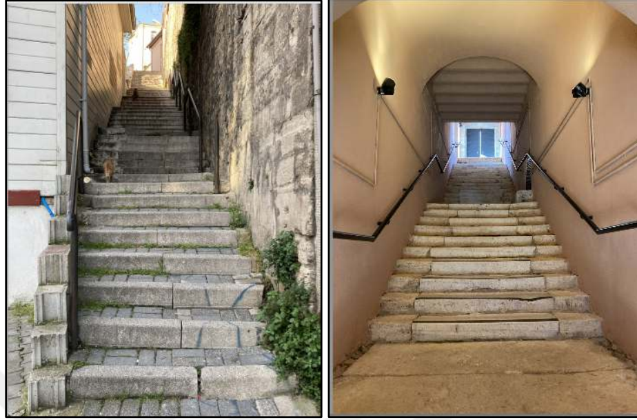
Figure 2. 2: The stairs connecting Helvacı Ali Street to Kartal Baba Street.
