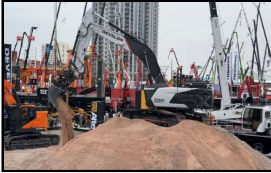
Figure 3.5: The Grab Excavator Considered as A Case Study in This Thesis [80].
