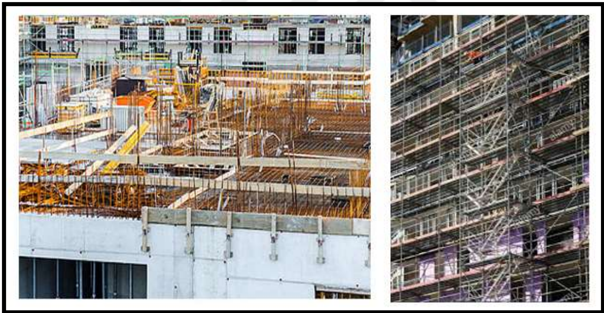
Figure 1.1: Examples of Large-Scale Construction Projects [1].
