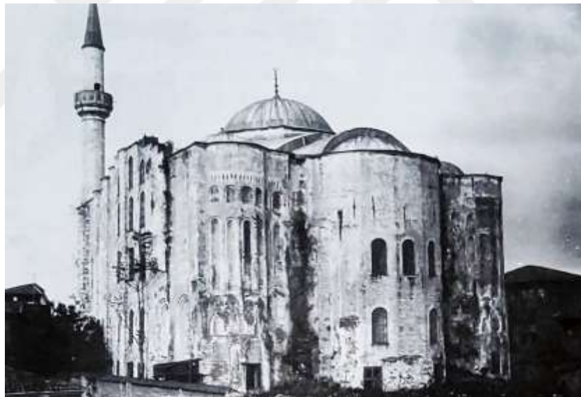
Figure 24: The atrium and exterior walls of The Church of St. Theodosia (Gül Cami) (From Marinis)
