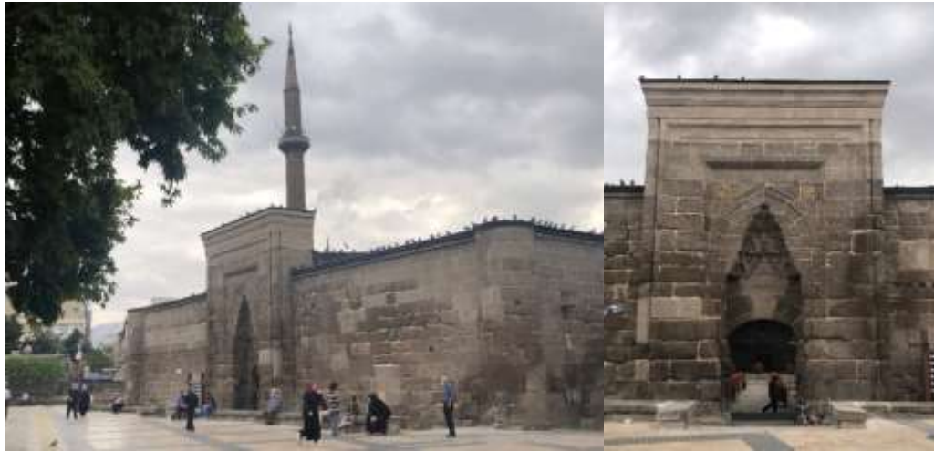
Figure 93: The exterior walls and portal of Hunad Hatun Madrasah (Photograph taken by the author)
