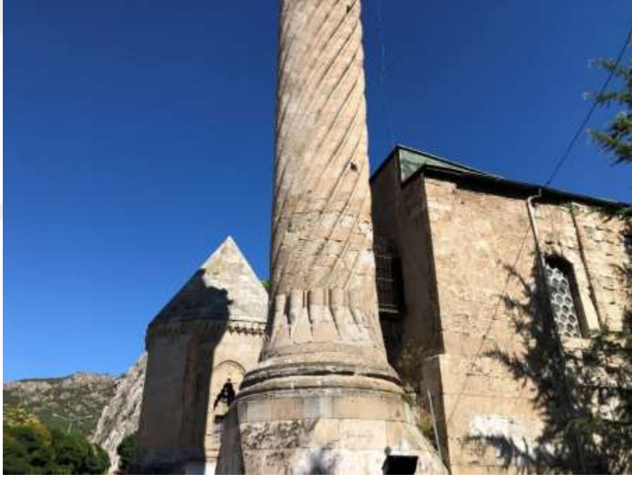
Figure 80: The exterior walls of Burmalı Minare Mosque (Photograph taken by the author)
