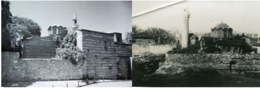
Figure 30: The atrium and exterior walls of Church of Theodore (Vefa Kilise Cami) (From Marinis and Paspates)
