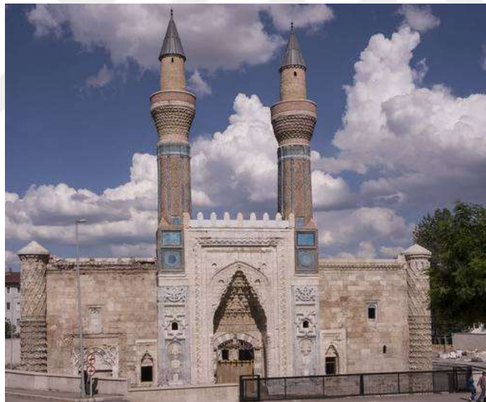
Figure 90: The exterior walls and portal of Gökmedrese in Sivas (From https://archnet.org/sites/2084/ )
