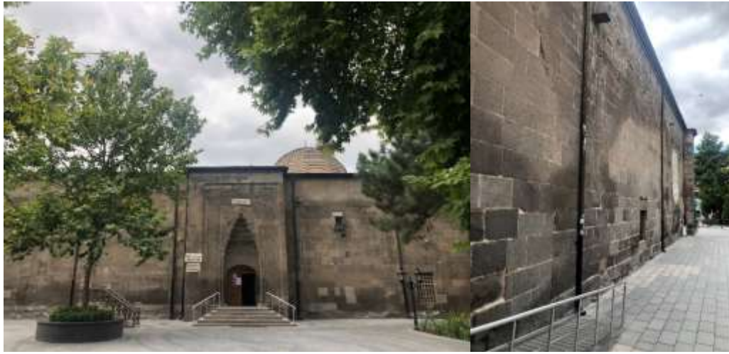
Figure 81: The exterior walls and portal of Hunad Hatun Mosque (Photograph taken by the author)
