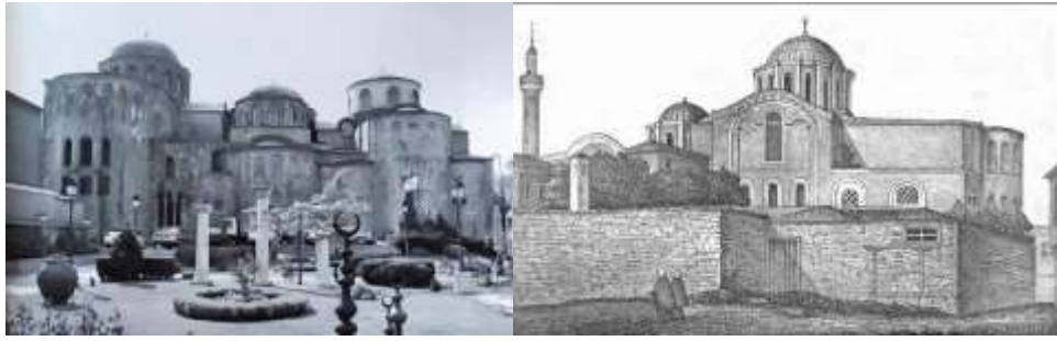
Figure 27: The atrium and exterior walls of the church of the Monastery of Pantocrator (Zeyrek Cami) (From Marinis and Paspates)
