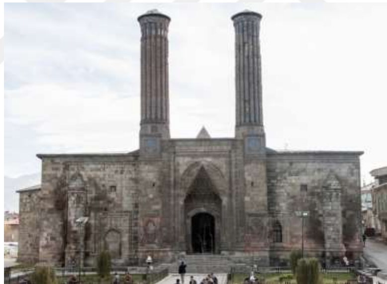
Figure 88: The exterior walls and portal of Çifte Minareli Madrasah in Erzurum (From https://archnet.org/sites/1947/media_contents/128020 )
