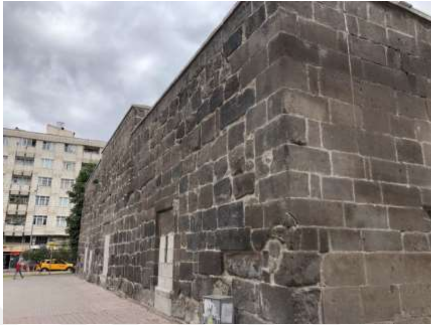
Figure 91: The exterior walls of Sahabiye Madrasah (Photograph taken by the author)
