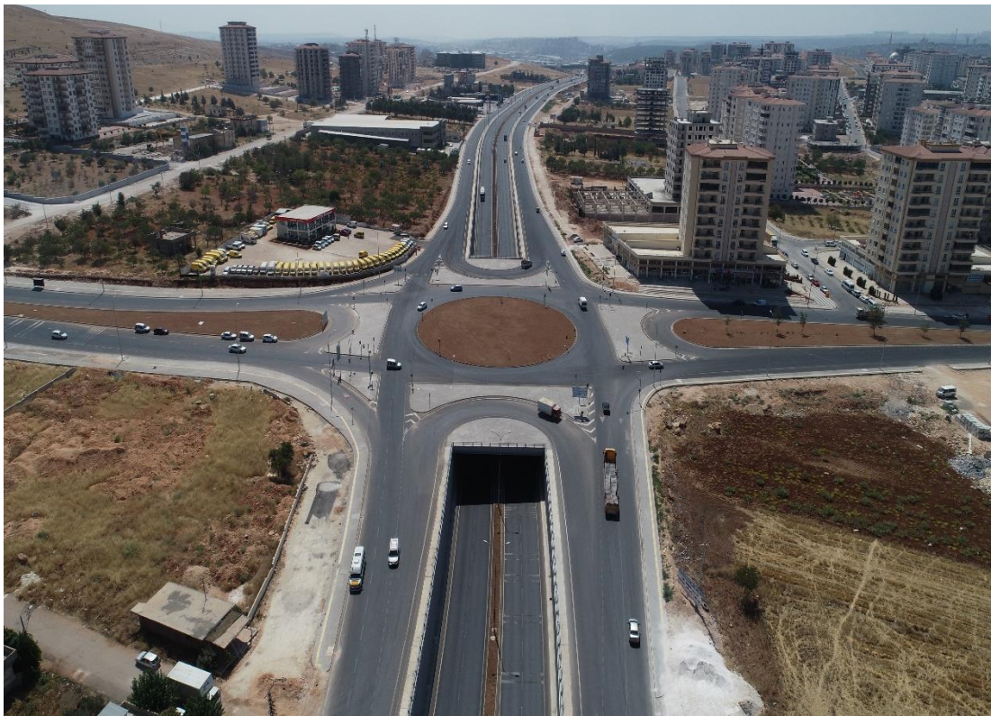
Figure 3.5: Beykent Bridge Crossing-1, Gaziantep, Turkey
