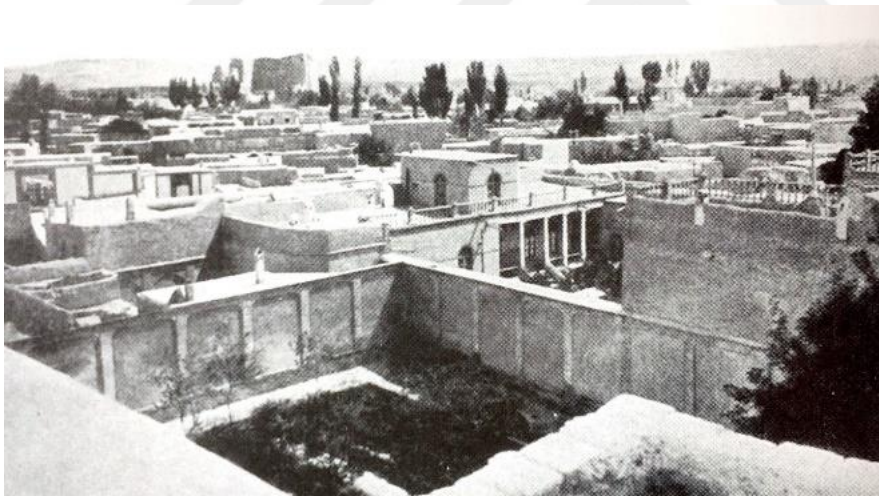
Figure 3.27 A view from courtyard houses in the early Pahlavi era, Tabriz Source: Pour Hossein, 2011, Historical sites and buildings of Tabriz
