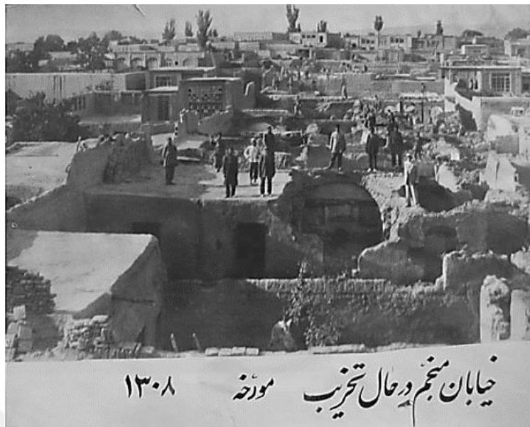
Figure 4.9. Destruction of historical district to construct Monajjem Street, Tabriz, 1929
