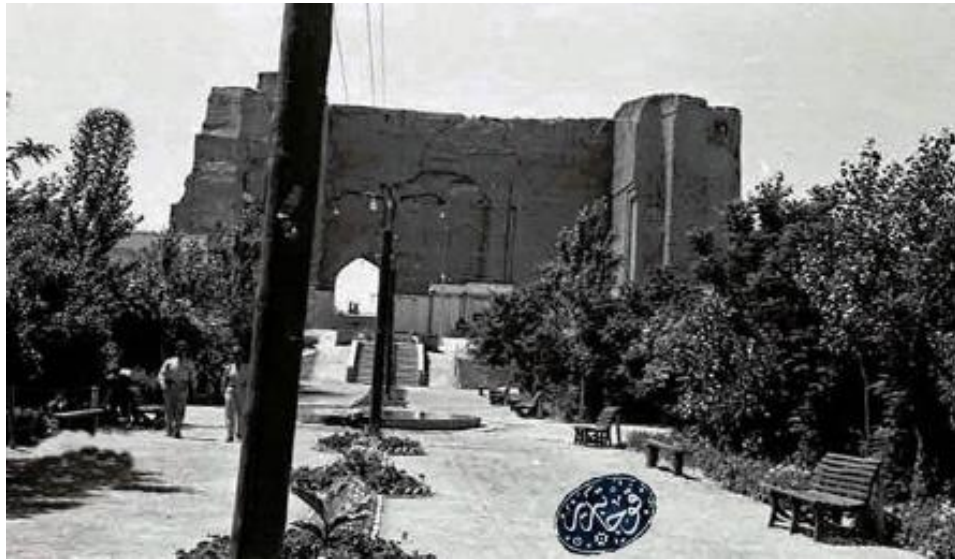
Figure 4.19 Bagh-e Melli, and Alishah Citadel, 1935
