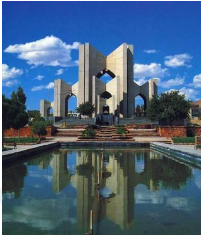
Figure 4.40 A view from ‘Maghbarat Ol-Shoara’
