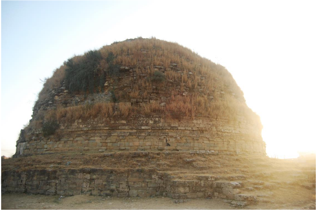
Figure 12. Parts of the Mankiala stupa's structure has been destroyed as a result of looting.
