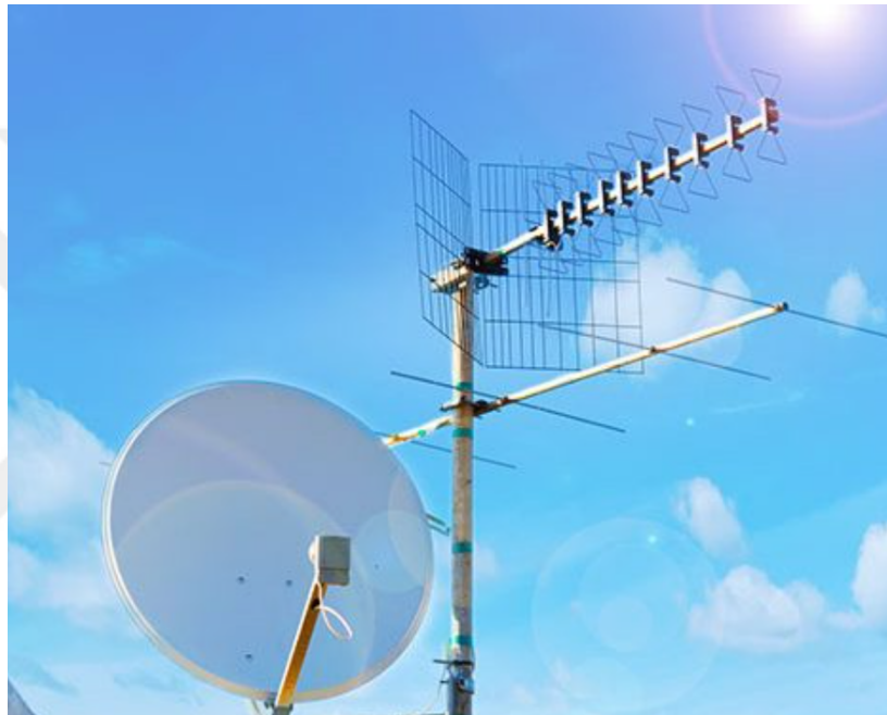
Figure 2.1: Low Noise Block Downconverter component in antennas
