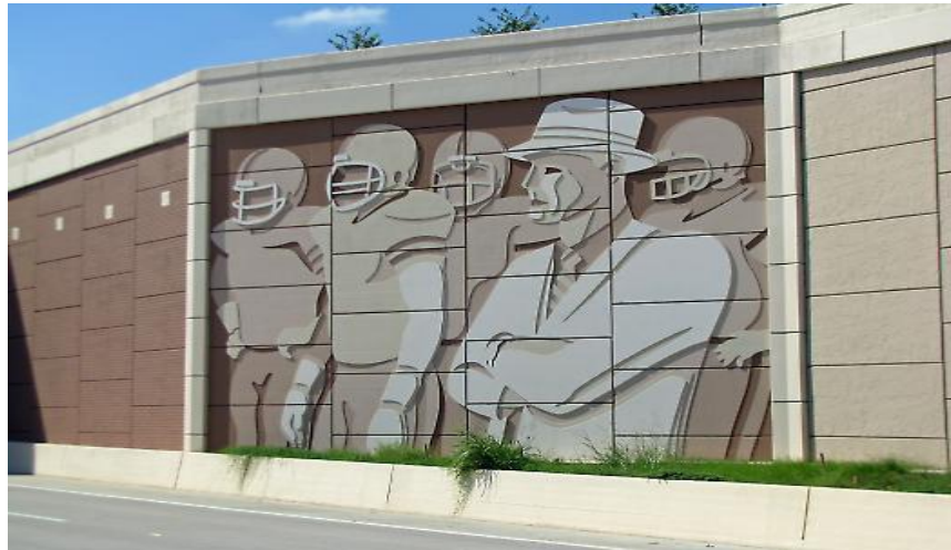
Figure 2.5 Facing element of MSE walls ( http://www.reinforcedearth.com )
