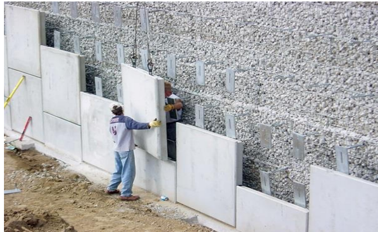
Figure 2.10 Post construction Facing ( http:// www.tensarcorp.com )
