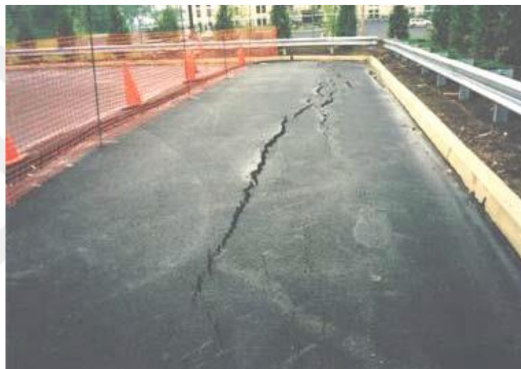
Figure 2.26 Tension cracks occurring exactly at the end of the wall reinforcement (Koerner and Koerner, 2012)
