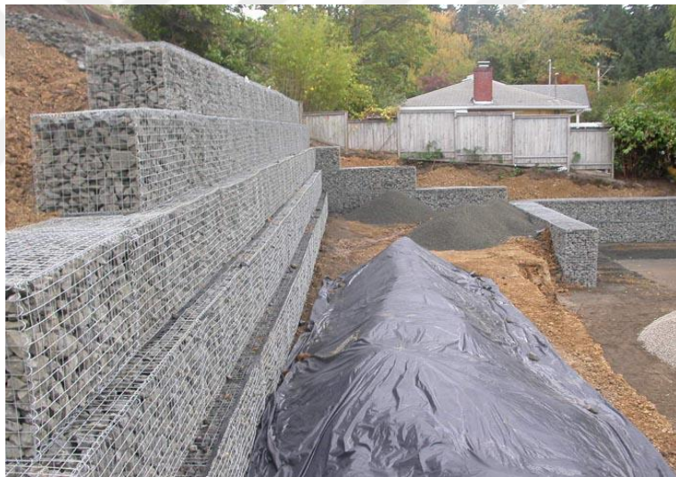
Figure 2. 9 Gabion Facing ( http://www.kaengineers.com )
