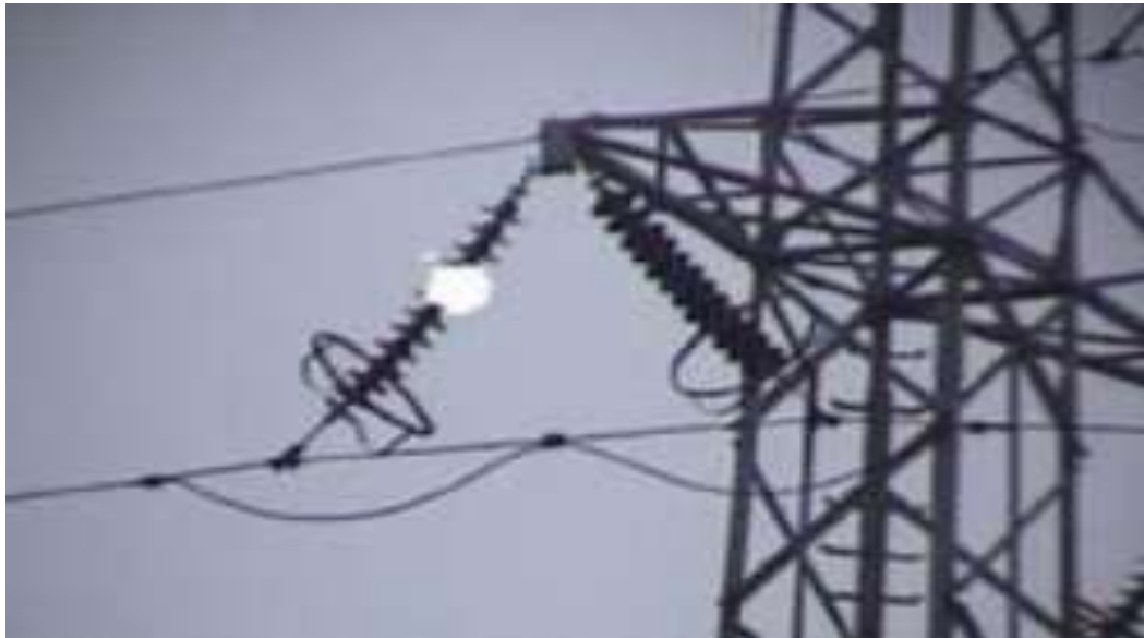
Figure.2.2: Corona effect on power lines [7]
