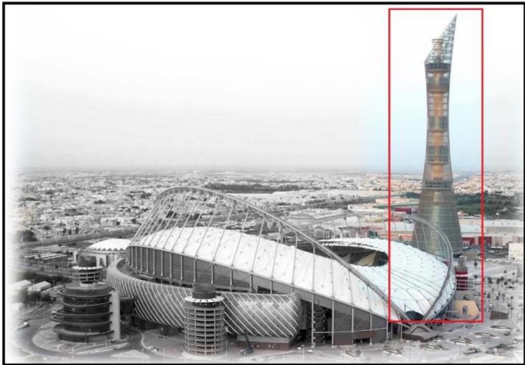
Figure 3.13: Wind Tower at Khalifa International Stadium (Nessim et al.,2023).
