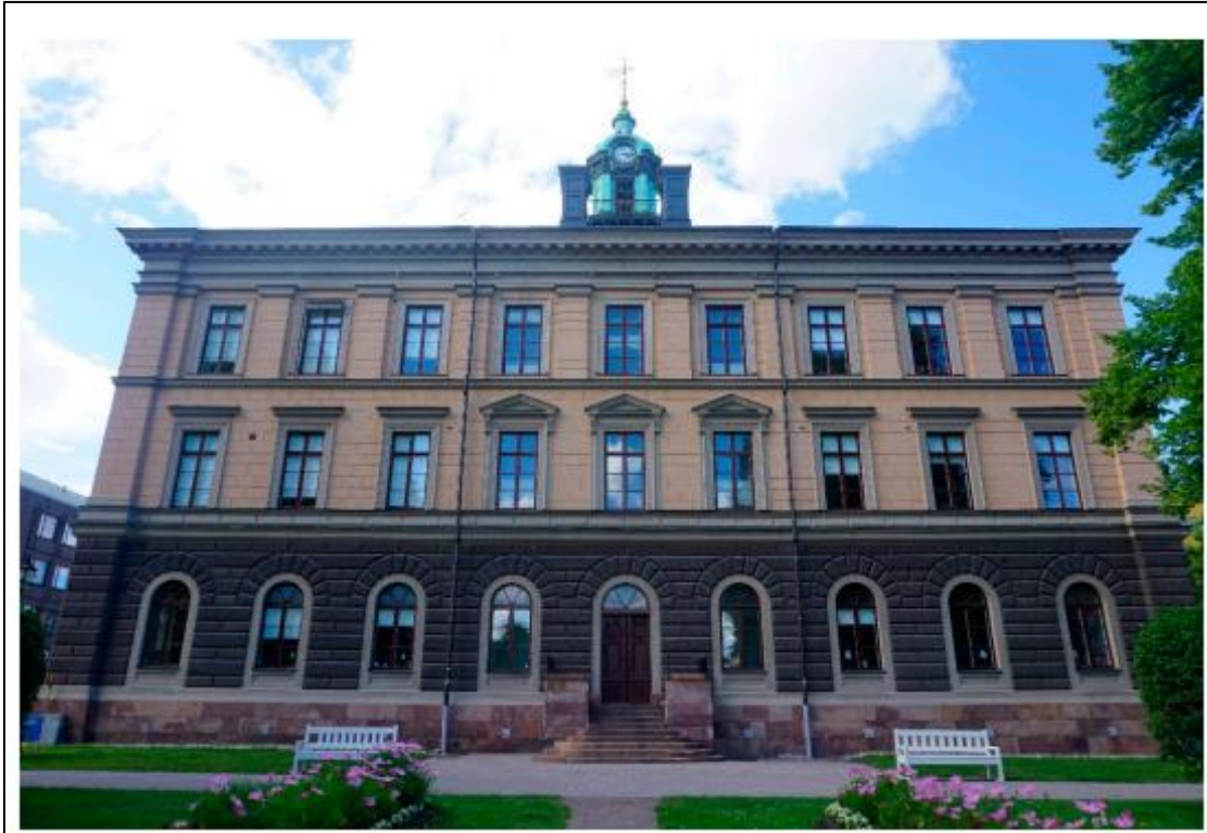
Figure 2.1: The Building of the City Hall of G, Bakhtiari, et al. (2020).
