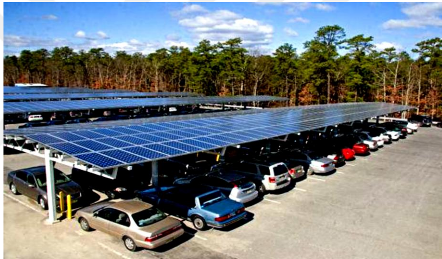
Figure 1.2 Richard Stockton School in New Jersey has solar umbrellas with a combined generating capacity of 2.1 megawatts that are powered by the arrays.
