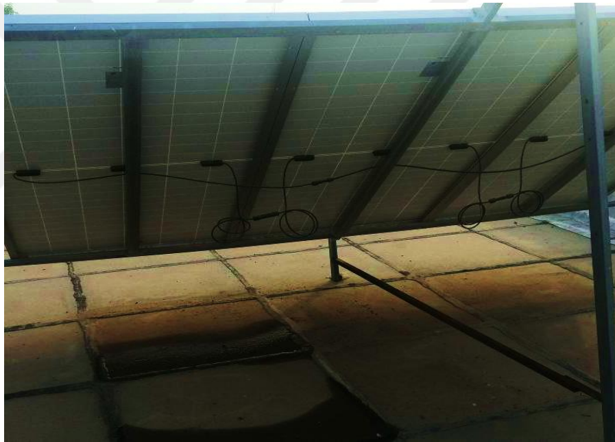
Figure 4.2 Solar panel (360 W) of each panel (Back side)
