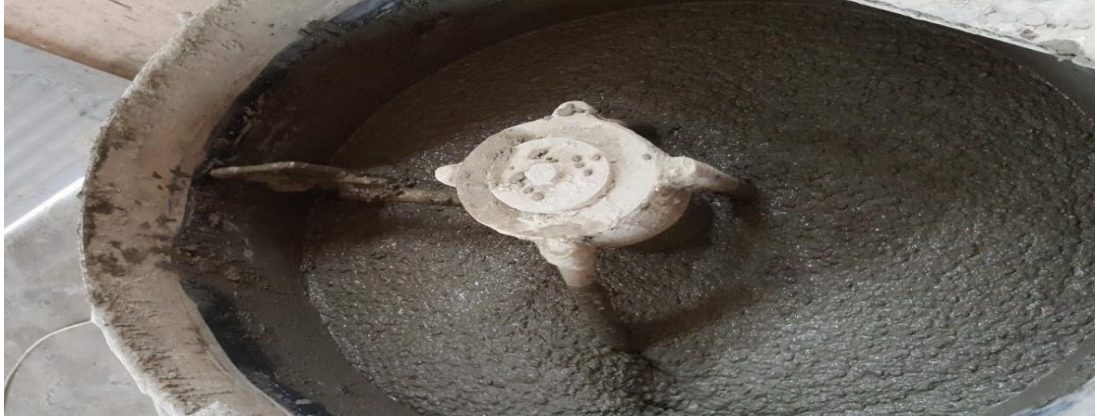
Figure 3.1 Mixing of the SCC.
