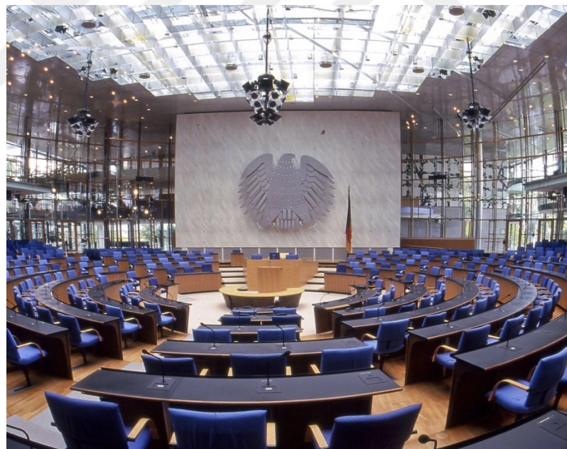
Figure 5. Acrylic glass micro-perforated panels (MPPs) installed in the plenum of Bonn Parliament Building, Germany (Fuchs & Zha, 1997)
