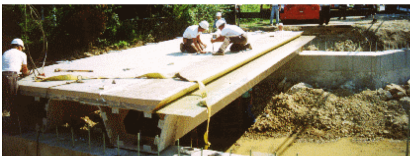
Figure 2.9 An epoxy/glass fiber-reinforced construction of a bridge. (www.bceo.org, 2008)
