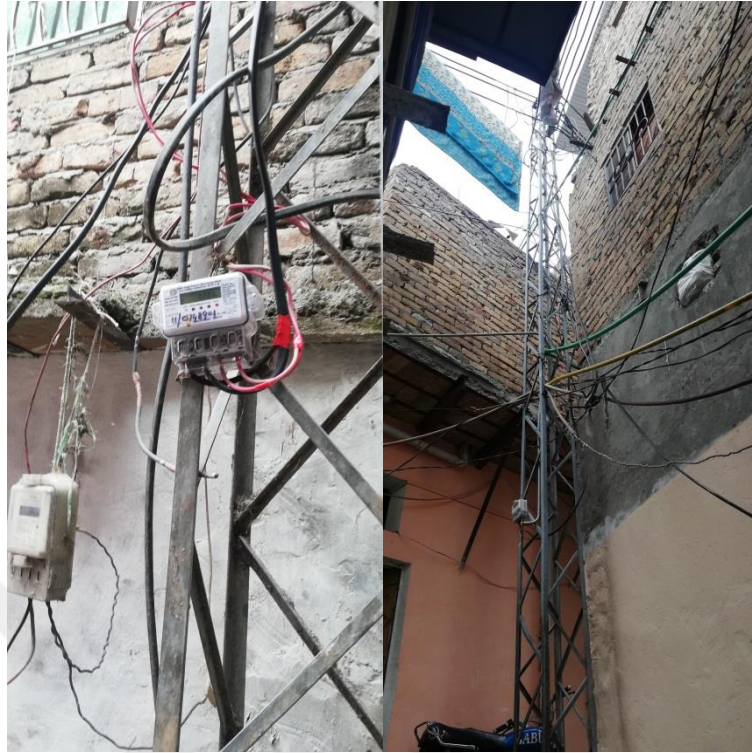
Figure 5.12: Precarious wires hanging from the main connection showing the extra wires added for temporal supply
