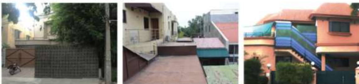
b. Images showing typical informal additions to the domestic space of Middle Class Houses. In Samanabad a house owner has occupied the outdoor building line setback through fencing making it part of the indoor garage space (Left); In Model Town side-setbacks have been consumed through informal additions to the service areas such as kitchen and laundry (Center); In DHA a house-owner has informally turned stair railing into a fence wall to prevent viewability of domestic space from the street (Right).
