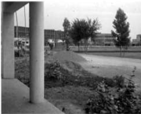
a. A photograph of Liberty Market (c. 1960's) showing under-construction standardized commercial buildings with ground level arcade and a central green space. From Naz & Anjum (2007).
