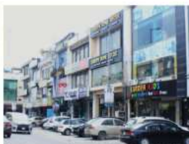
b. Commercial area with controlled building activity and formal public-private interface
