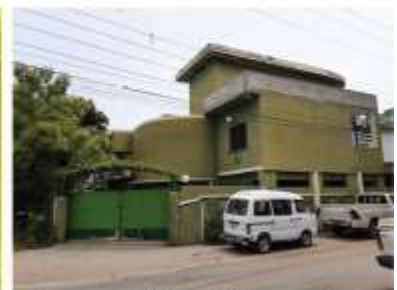
c. Incremental floor additions and set-back violation in residential blocks with mid-range lot sizes.
