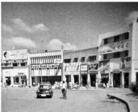
c. A photograph of Main Market Gulberg 2(c. 1960's) showing privately developed modern commercial buildings with ground level arcade surrounding a vehicular space.
