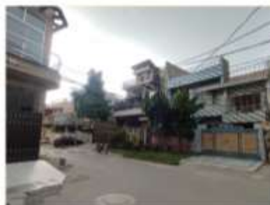
a. Typical residential architecture of improvement and upgradation
