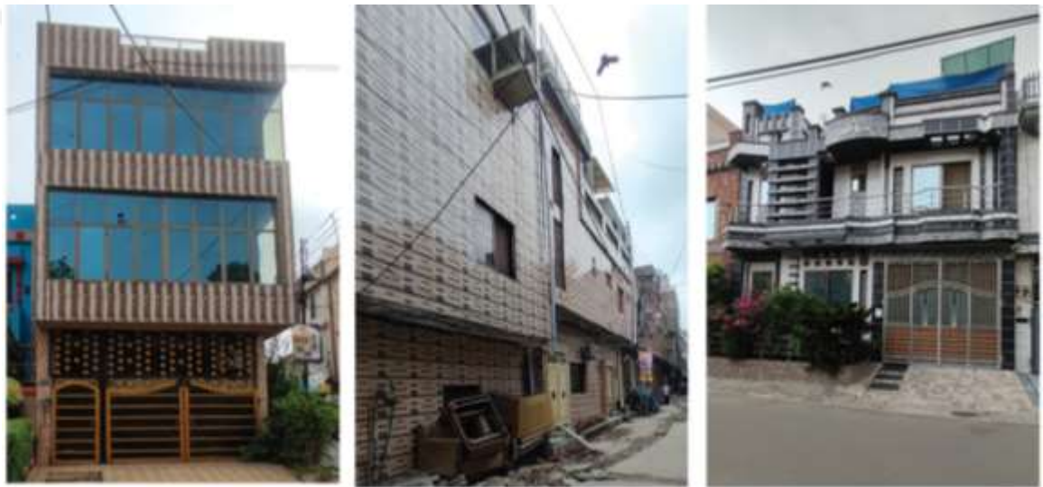
A house in Samanabad is informally converted into a commercial office space utilizing glazing and glazed tile work (Left); An informal rental apartment building in Kanal Park, Gulberg with monolithic facade-uplift by a local developer (Center); A developer constructed house in Samanabad with ornamental facade-work and tinted glass aluminium windows.
