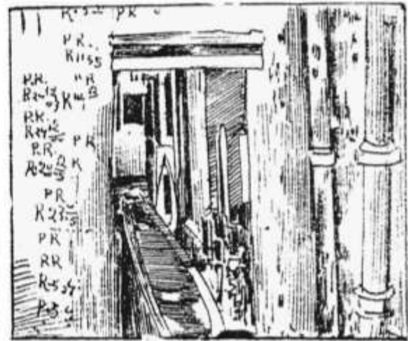
b. An 1890 illustration showing unsanitary conditions in a dark and damp gali with drain and sewage pipes running along the wall and the other wall shows the municipal chalkings recording the number of rats culled.
