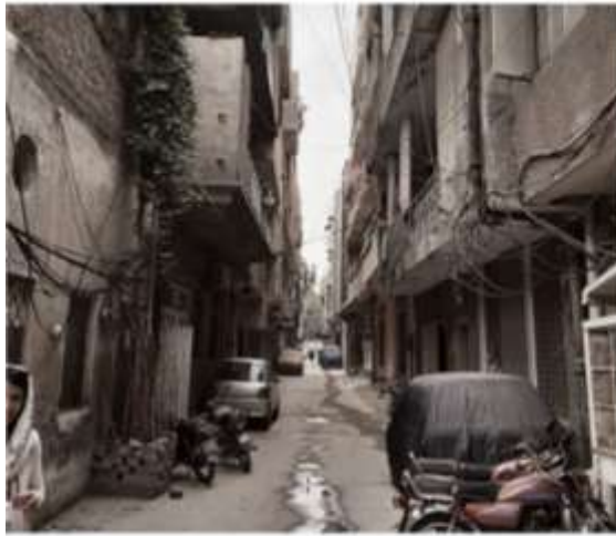
a. A typical street showing overtime vertical addition of 3 to 4 floors per dwelling with set forwards and set aboves protruding onto the street for maximization of slab footprint.
