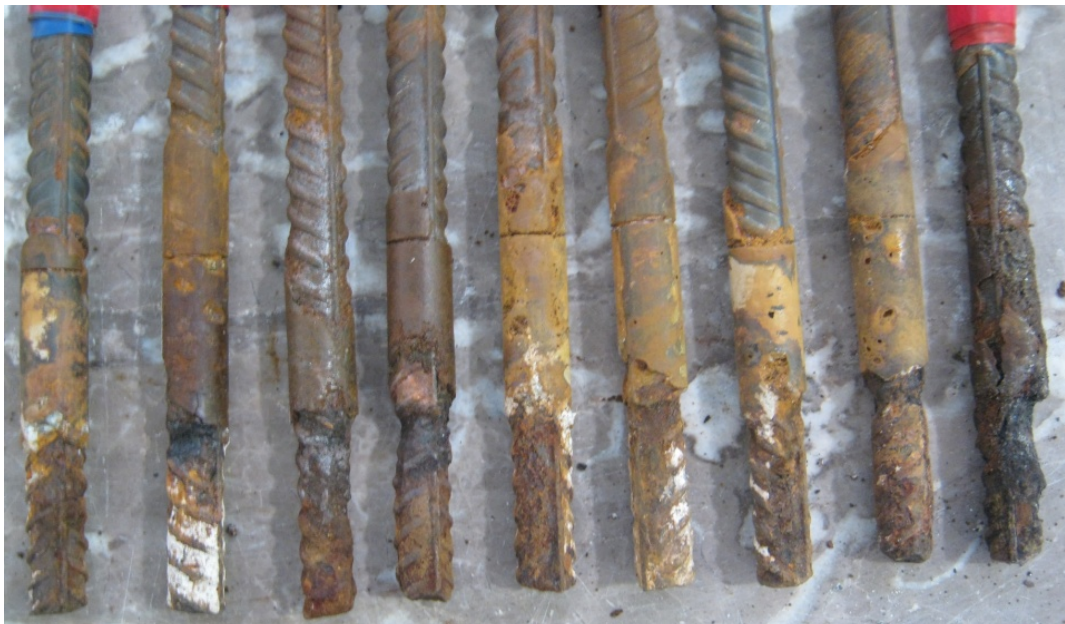
Figure 5.1: Before cleaning of reinforcement bars.
