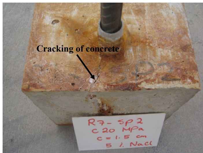
Figure 5.8: Recorded maximum crack width with a w/c ratio of 0.75 for the lowest c/D ratio.
