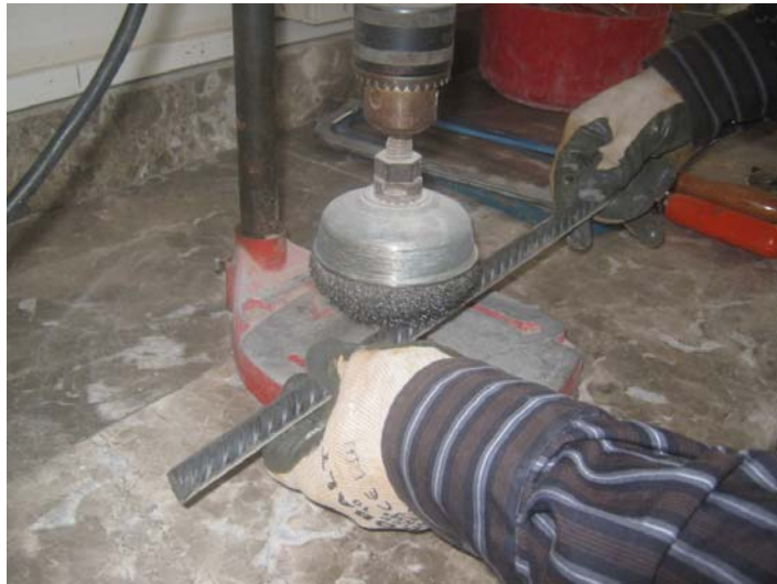
Figure 4.12: Cleaning surface of reinforcement bars.
