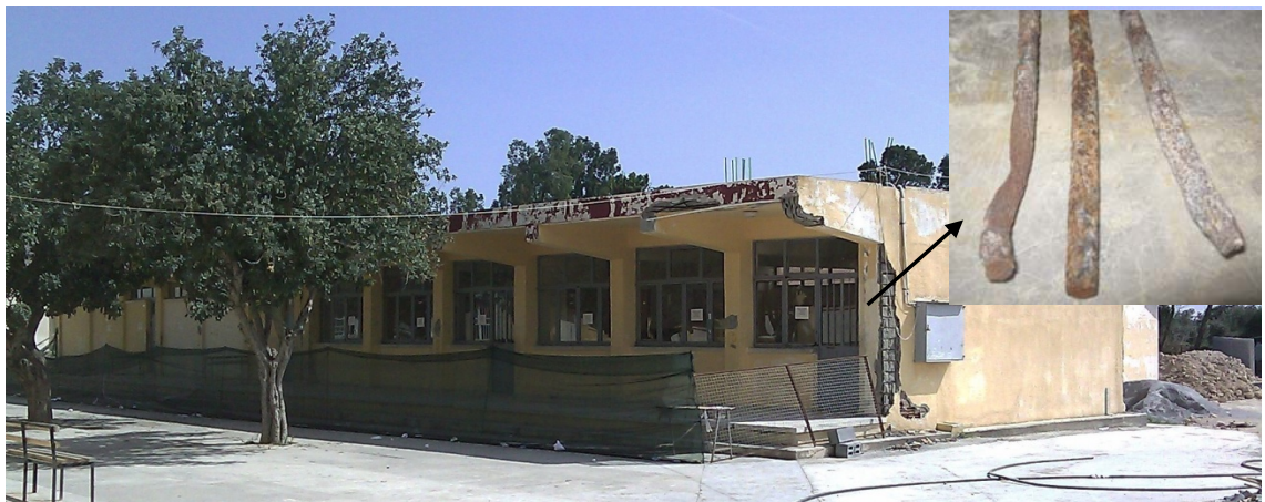
Figure 3.38: Analyzed high school building.
