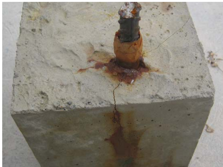
Figure 4.41: Volumetric expansion of a corroded reinforcement bar.
