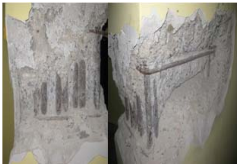
Figure 3.20: Inside face of S 3 column.
