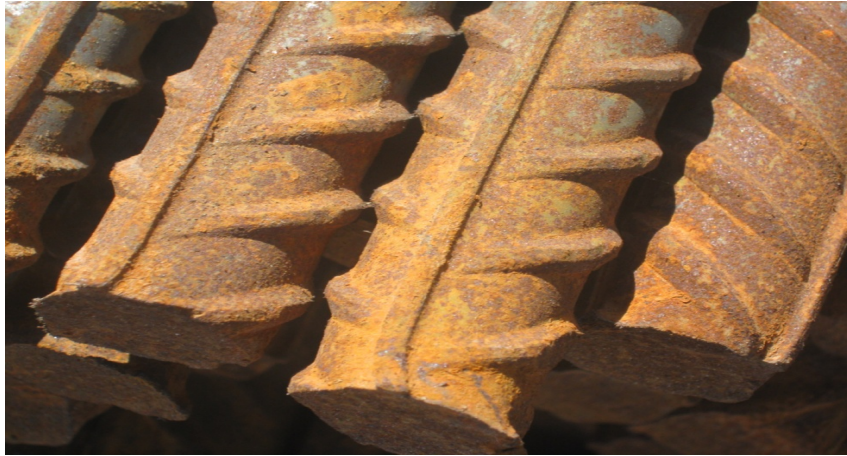
Figure 4.2: General condition of reinforcement bars in the market of Famagusta.
