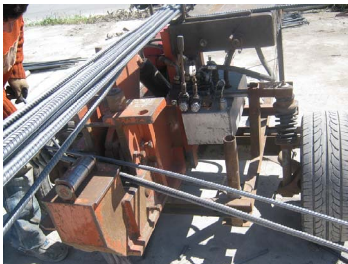
Figure 4.4: Cutting of reinforcement bars.
