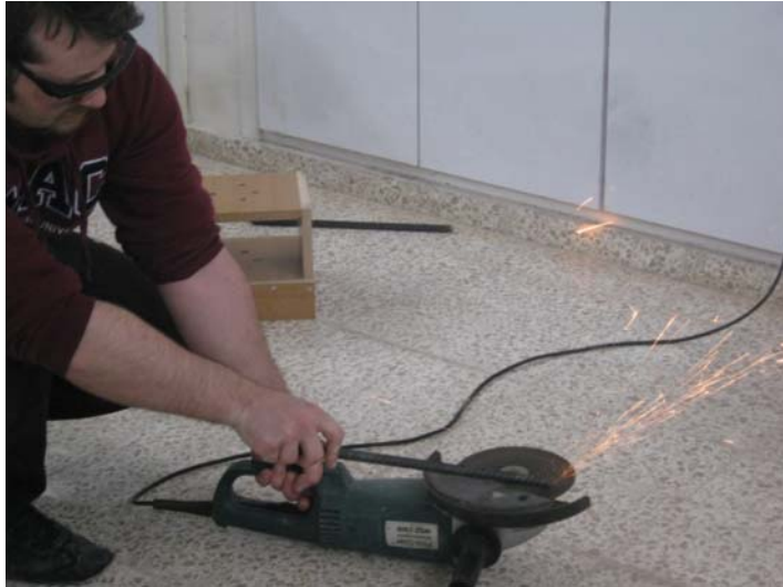
Figure 4.30: Smoothing the edge of reinforcement bars.
