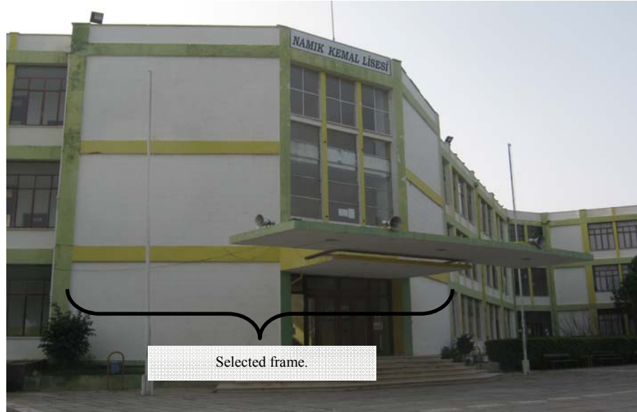
Figure 3.17: Analysed high school building.
