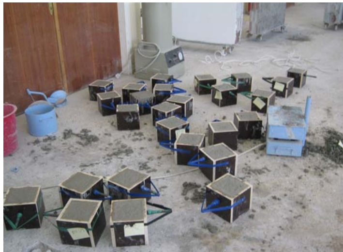
Figure 4.53: Second group of concrete specimens ( w/c= 0.40 ) after casting concrete.
