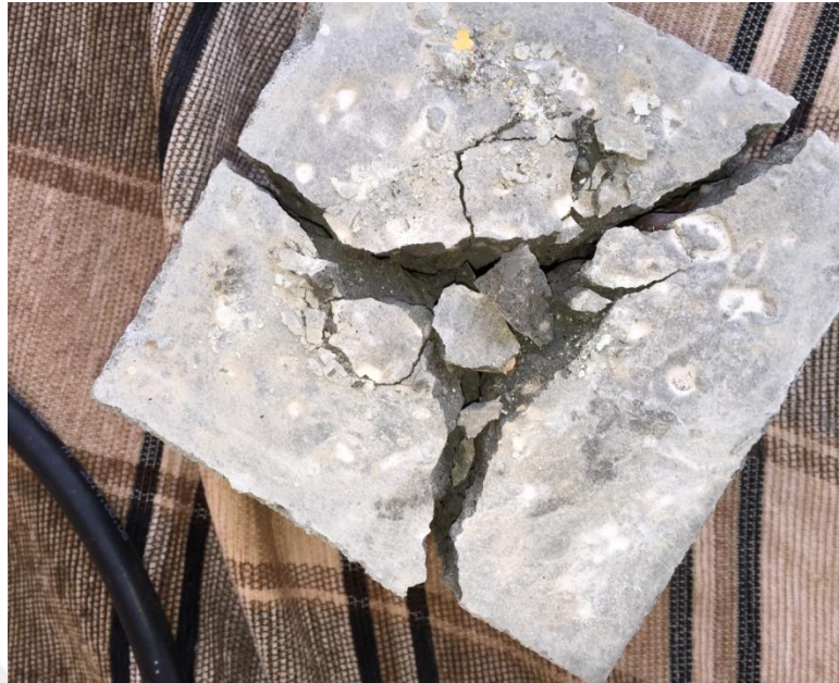
fig(3.18) failure concrete
