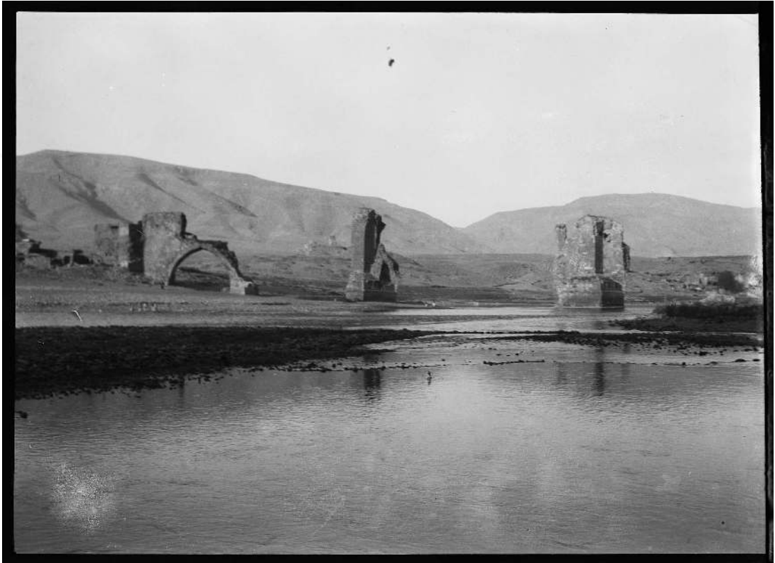
Figure 3.11. The Remains of the Hisn Kayfa Bridge, Photo by Albert Gabriel, 1908-34, AG20K004188, Albert Gabriel Fund INHA, Media Library of Architecture and Heritage, France (POP-Plateforme Ouverte du Patrimoine).
