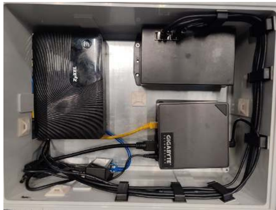
Figure 3.7: An exemplary electrical panel.
