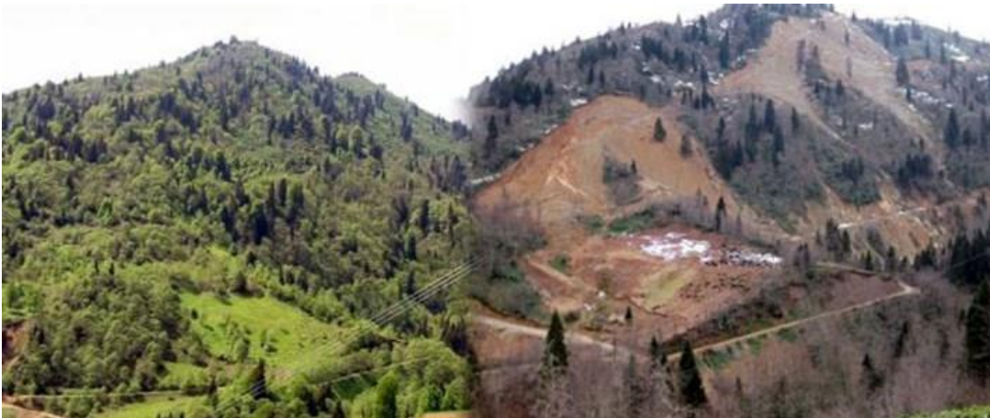
Figure 11: Environmental Destruction Caused by HEPP Construction, Before and After Source: NTV , 2011
