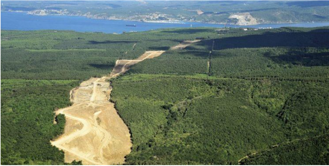
Figure 10: Environmental Destruction Caused by the Third Bridge and Connection Roads Source: Gazete Yolculuk , 2018
