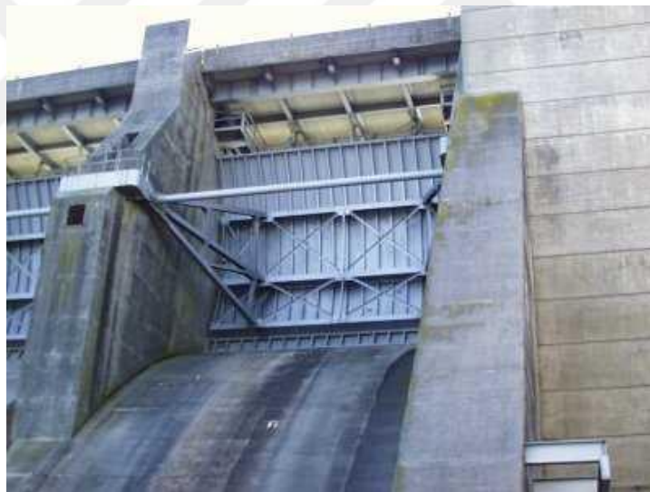
Figure 1.1 Radial Gate of John H. Kerr Dam (Source: Wikipedia)
